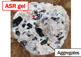
Coring sample of concrete
