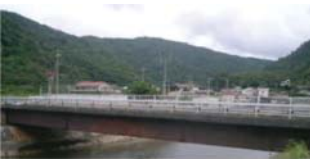
-bridge Full view-
