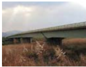
Complete view of the bridge
