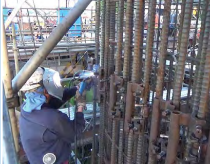
34. Enclosed Welding of Pier Re-bar
