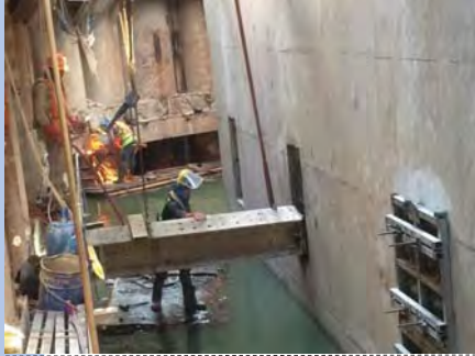
40. Removal of Struts and Wales
