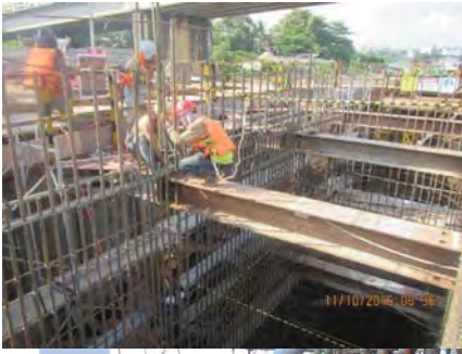
33. Pier Re-bar Installation
