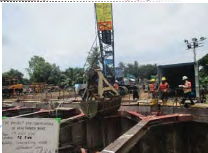
21. Laying Gravel Materials
