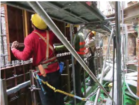
36~37. Formwork Installation and Concrete Casting for Pier
