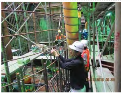
35. Ultrasonic Flaw Detection Test of Enclosed Welding
