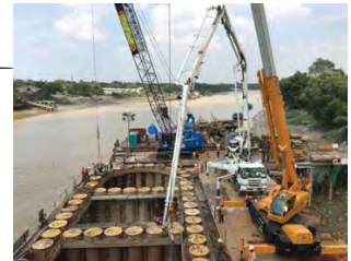
Concrete Filling inside SPSP (8000mm)
