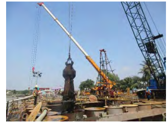
Excavation inside SPSP
