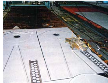
GAS Frame Cut
