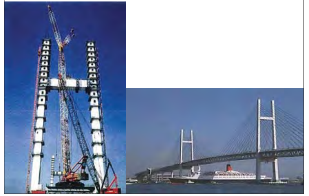
Crawler crane and tower crane
