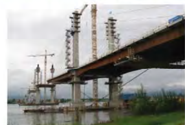
The Golden Ear Bridge at Vancouver (span:242m) PFI (German Company)
