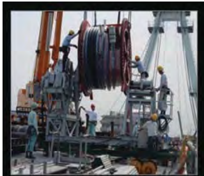
Reeled cable set to unreeler machine
