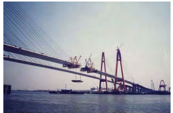
Cantilever construction
