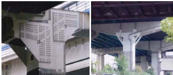
Repair by steel plate (bolting) Rigid frame type steel piers
