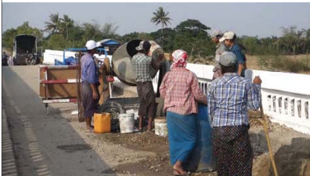
Repair work of the slabs, 11 th Dec., 2016 Mix proportion of concrete...???
