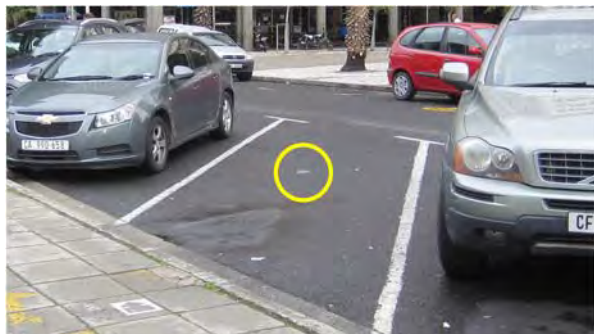
Embedded sensor on the center of parking slot
