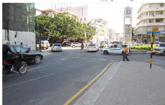
Widening of Roundabout for Providing Smooth Traffic
