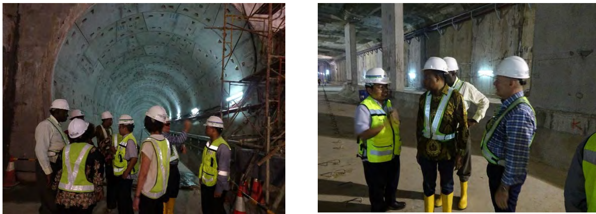
Photo 2.15 Site Visit of MRT Construction
