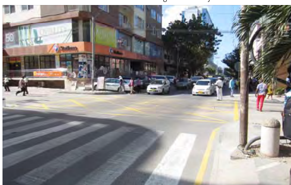
Yellow Box Marking at the Intersection of BRT Crossing
