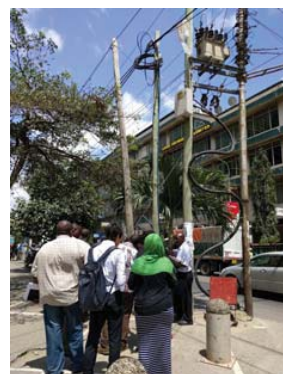
Joint Site Visit on 16 th Sep
