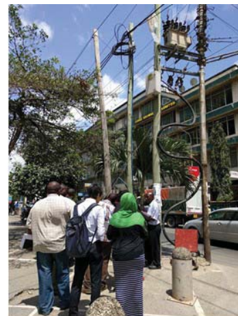
Joint Site Visit on 16 th Sep
