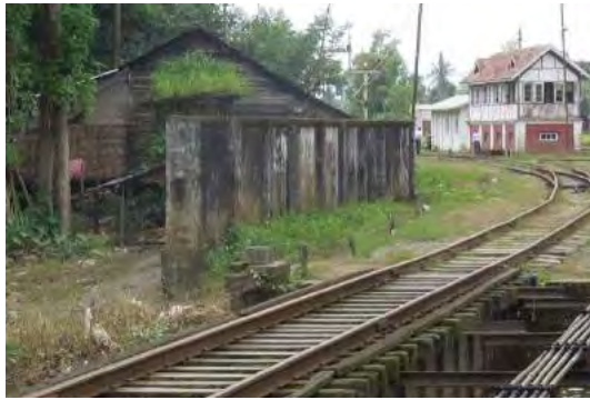
(a) Brick Wall Type Fence
