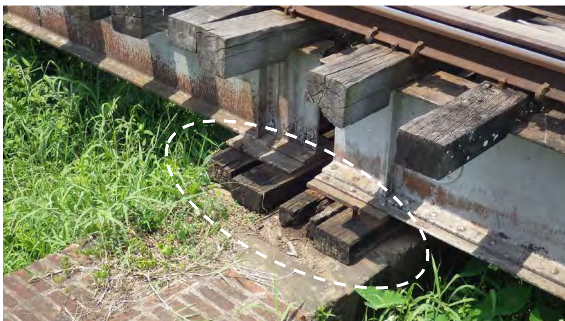
Figure 5.5.3 Unstable Shoe Structures (Bridge No.325)
