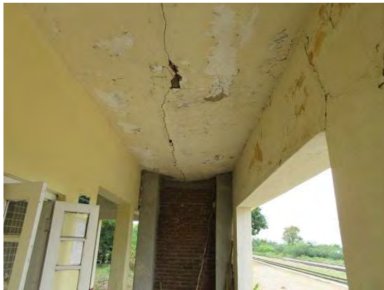
Figure 5.9.7 Ceiling collapse of Shanywa Station
