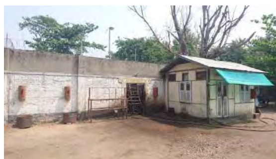
(b) Fuel Pump Room (Fueling Facility)
