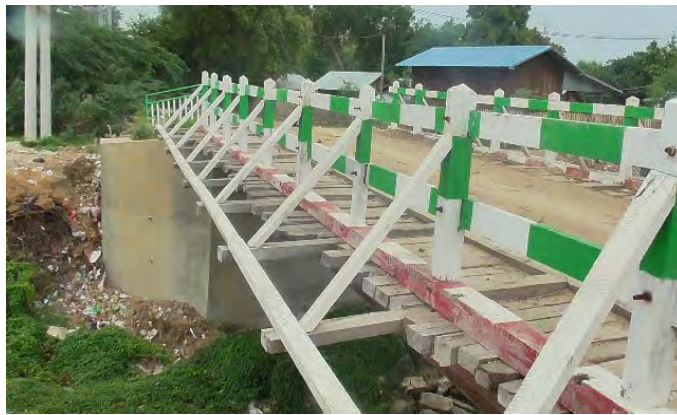
Figure 5.19.4 Existing Wooden Bridge
