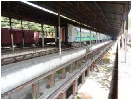
(a) Inspection Pit
