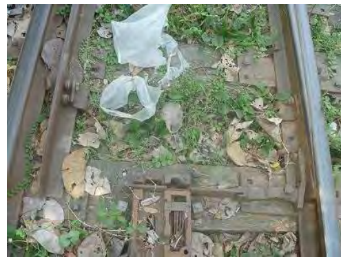
(b) Point Machine without Proper Maintenance
