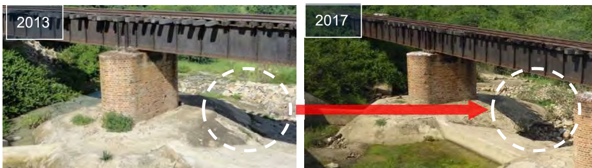
(a) Bridge No.588 (2013)
