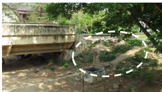
(a) Bridge No.393
