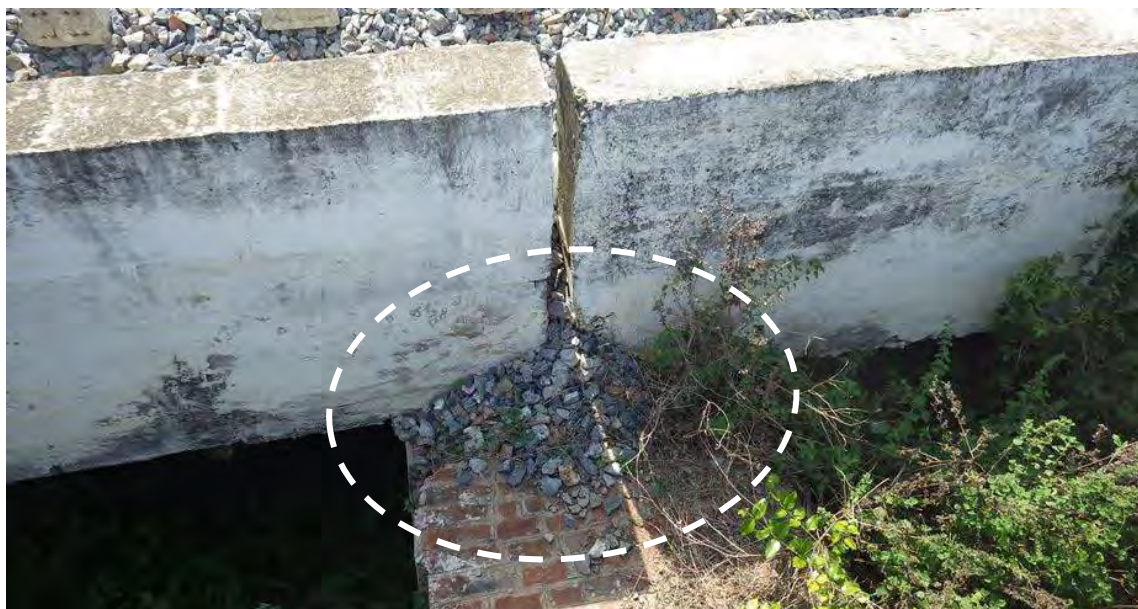
Figure 5.5.17 Spillage of Ballast from Joint Gaps between Girders (Bridge No.586)
