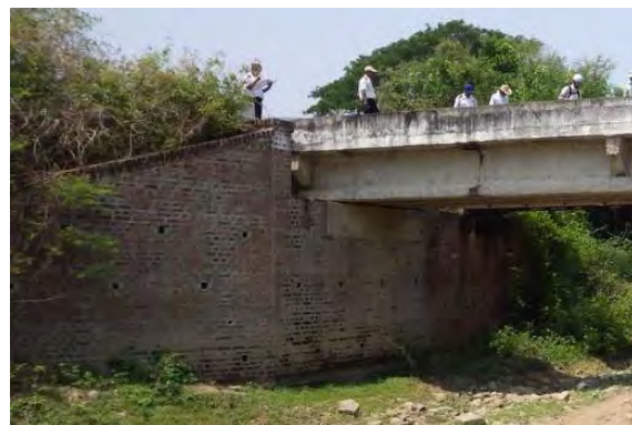
Brick - Wing Wall / Retaining Wall
