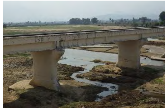
Reinforced Concrete Pier
