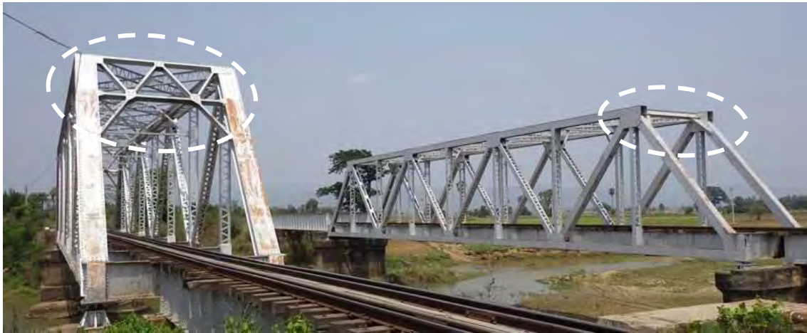
Figure 5.5.8 Interference with Portal Bracings to Construction Gauge (Bridge No.373)
