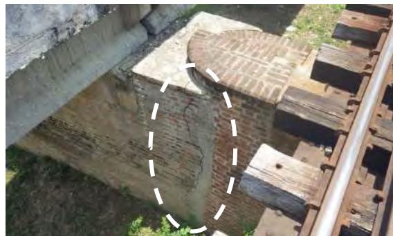
(c) Bridge No.519
