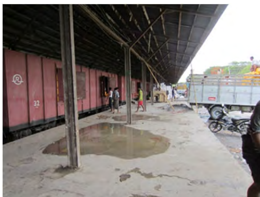
(a) Cargo Handling in the First Area
