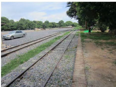
(a) Temporary Platform for Unloading Containers
