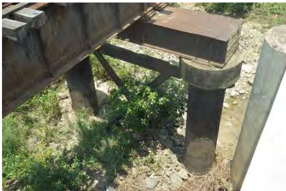
Concrete-filled Steel Tubular Pier
