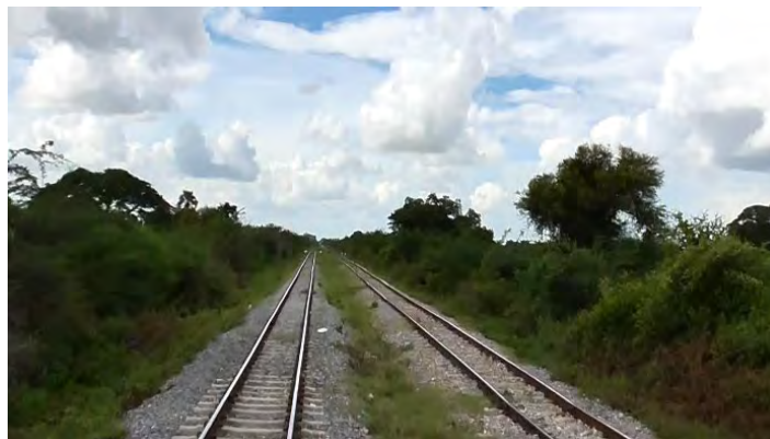
Figure 5.19.1 Existing condition of railway
