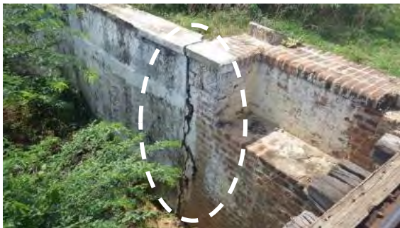
(a) Bridge No.497
