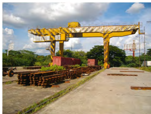
(b) Container Crane
