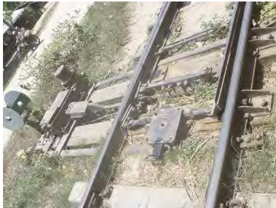
(a) Electric Point Machine and Key Lock
