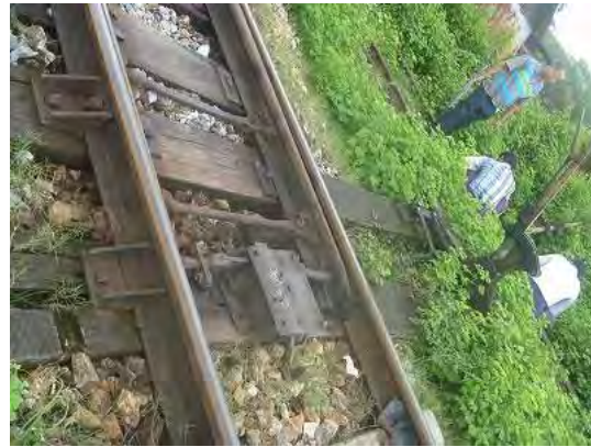
(b) Manual Point Machine (Key-interlock)
