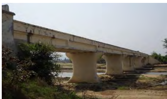
(a) Bridge No.453
