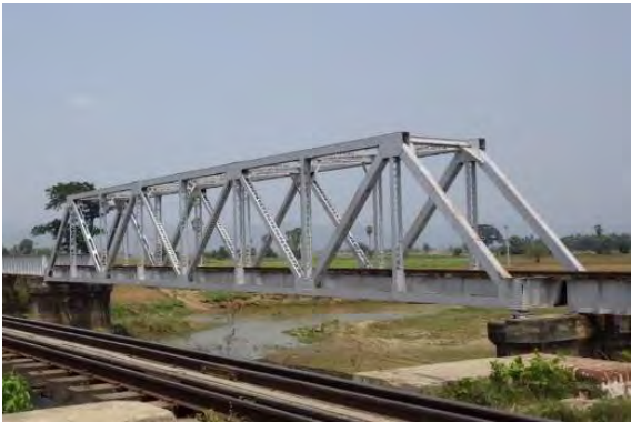
Steel Through Truss Girder
