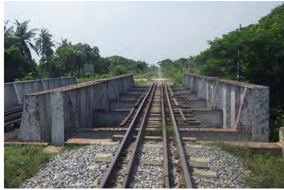
Steel Through Plate Girder
