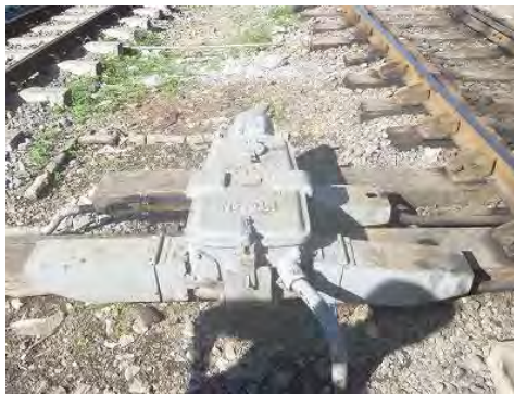
(c) Electric Point Machine (Mandalay)
