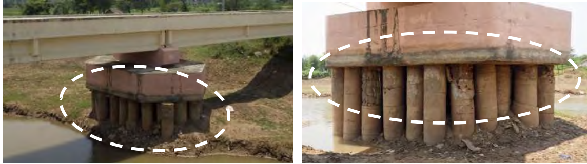
Figure 5.5.24 Damages of Pile Foundations (Bridge No.719)
