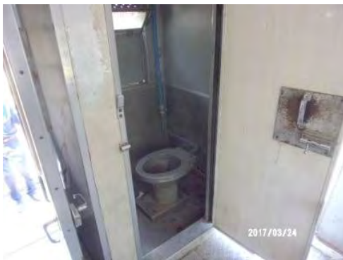
(c) Western-style Toilet
