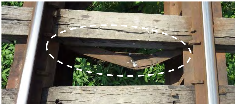
Figure 5.5.5 Deformation of Lateral Bracings under Tracks (Bridge No.384)
