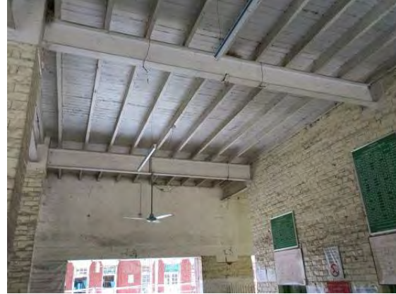
Figure 5.9.6 Steel structure of Tajee station
