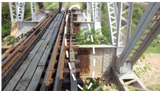
(a) Bridge No.453
