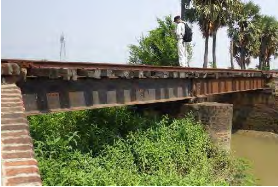
Steel Deck Plate Girder
