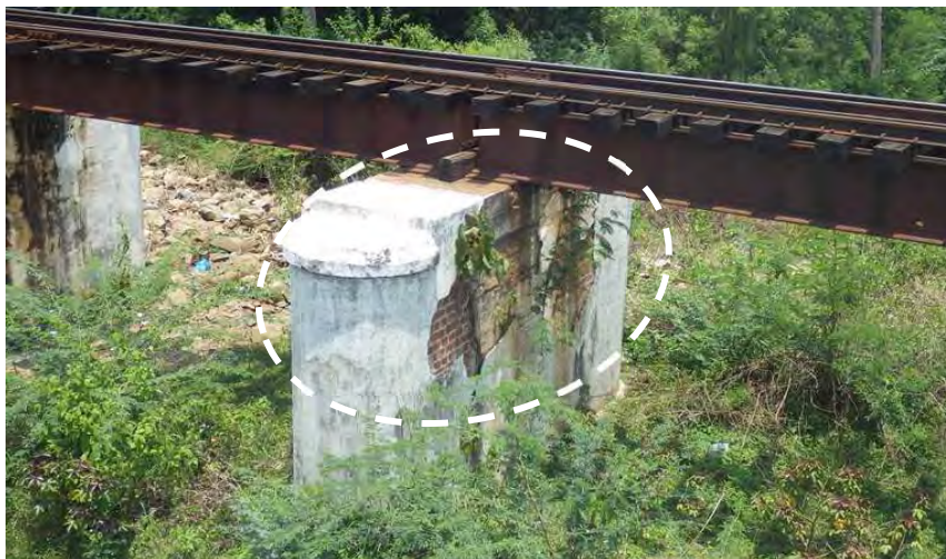
Figure 5.5.20 Surface Coating with Mortar (Bridge No.527)
