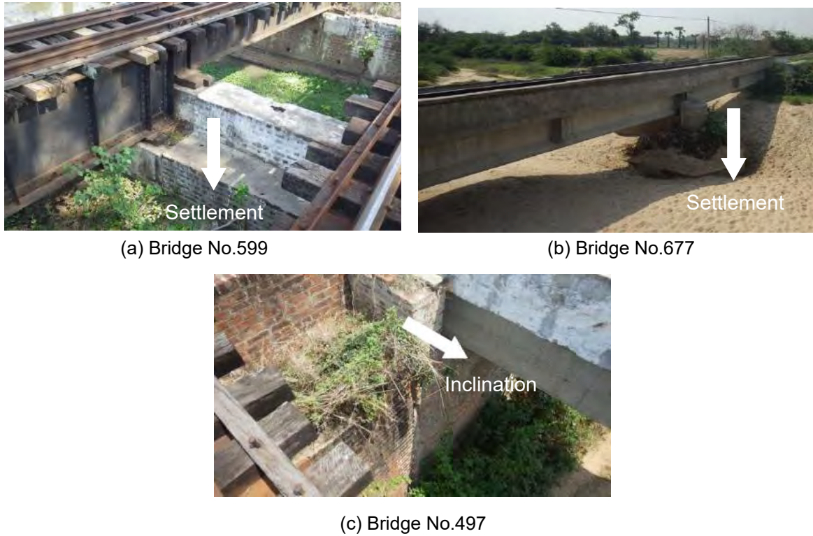
Figure 5.5.19 Structural Instability Due to Bearing Capacity Deficiency of Substructure Foundations
