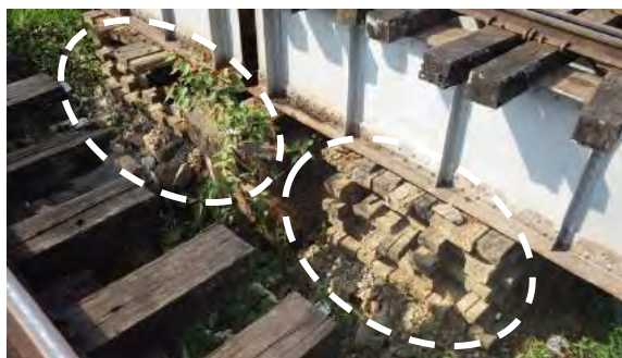
(a) Bridge No.270
