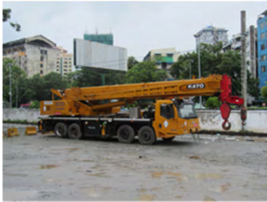
(a) Crane Used for Unloading Containers (Wadan Station)
