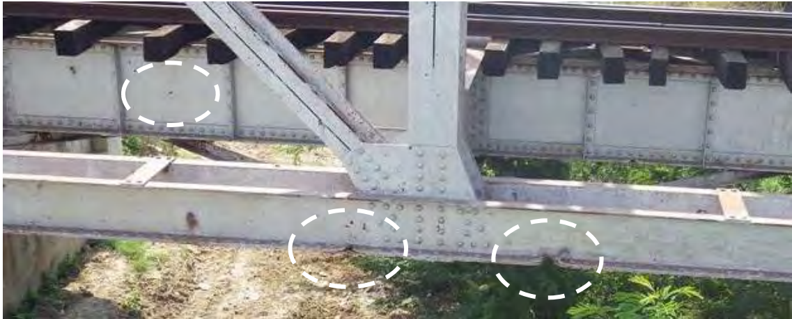
Figure 5.5.14 Damage of other Structural Members (Bridge No.683)
