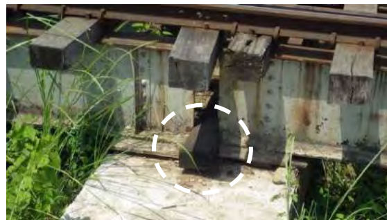
(c) Bridge No.320A
