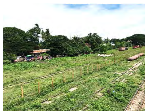
(b) Storage Track
