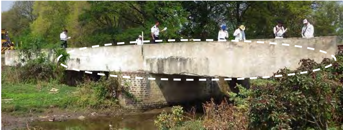
Figure 5.5.16 Girder Side Surface Covered with Repair Mortar (Bridge No.436)
