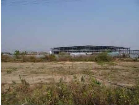
(a) Factory Appearance (Mar. 2017)
