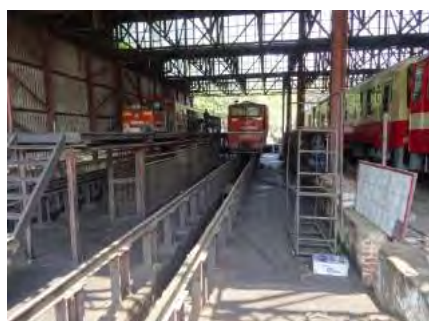
(a) Inspection Pit
