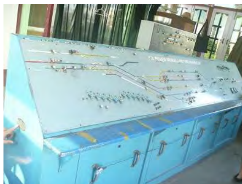
Figure 5.12.2 Interlocking Control Panel
