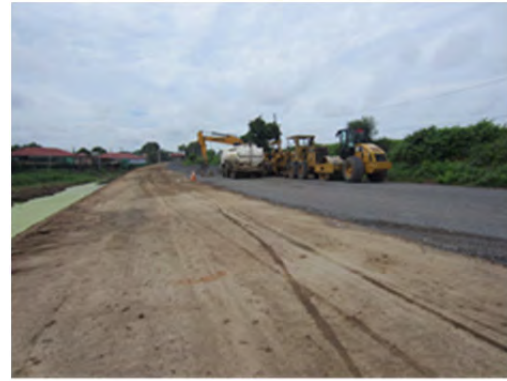
(b) Access Road
