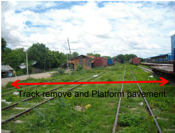
(a) Site where Cargo Handling Platform is to be Built
