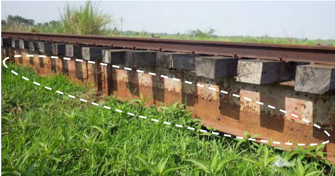
Figure 5.5.6 Corrosion due to Repeating Submergence (Bridge No.291)
