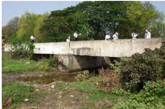
Reinforced Concrete Girder
