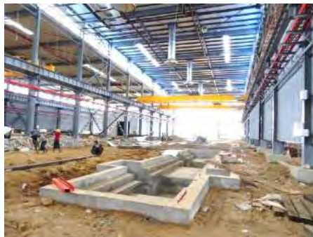
(c) Inside the Main Building 1 (Sep. 2017)
