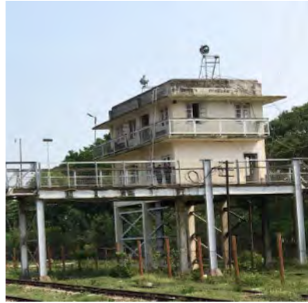
(b) Signal Cabin (Tower)
