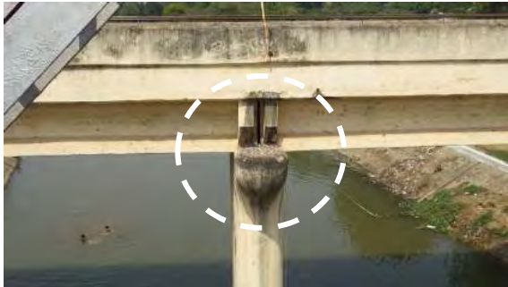
(a) Bridge No.393
