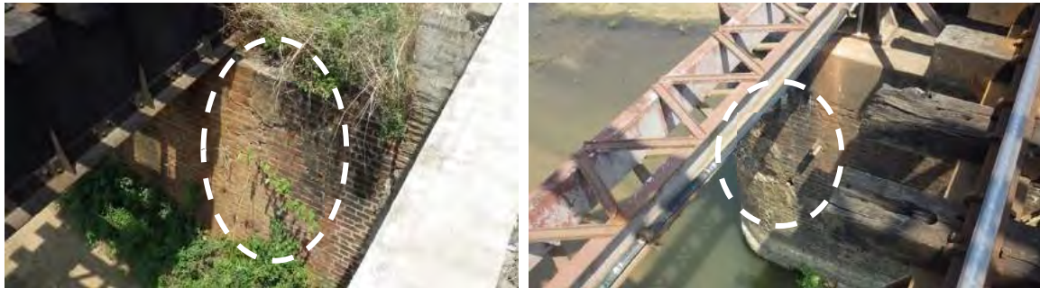
(a) Bridge No.497
