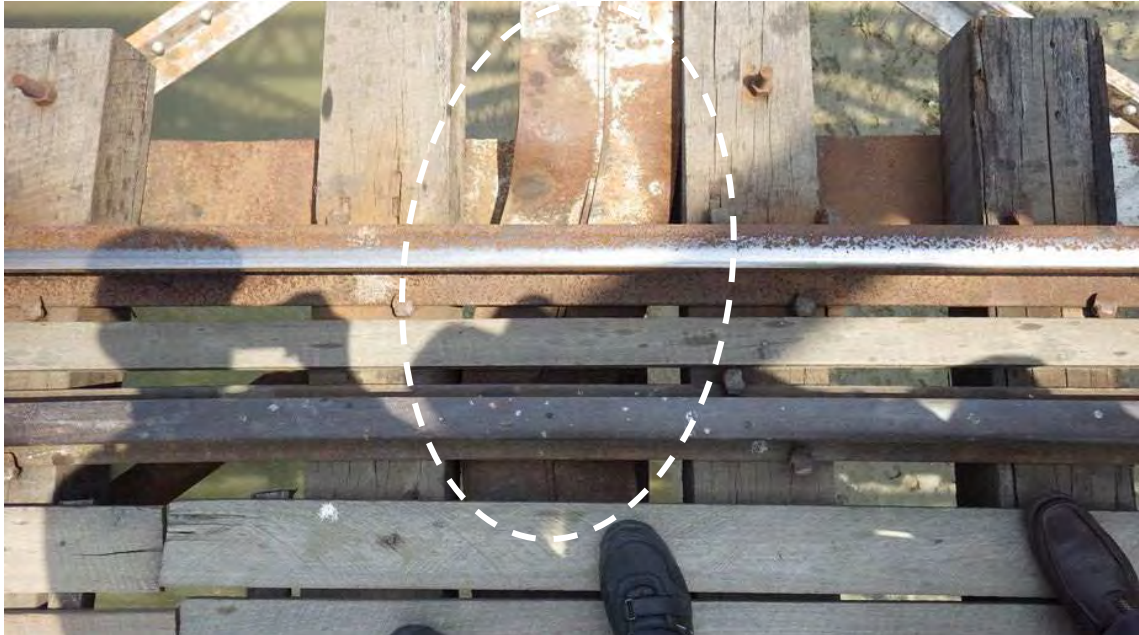
Figure 5.5.12 Deformation of Cross Beams under Tracks (Bridge No.373)
