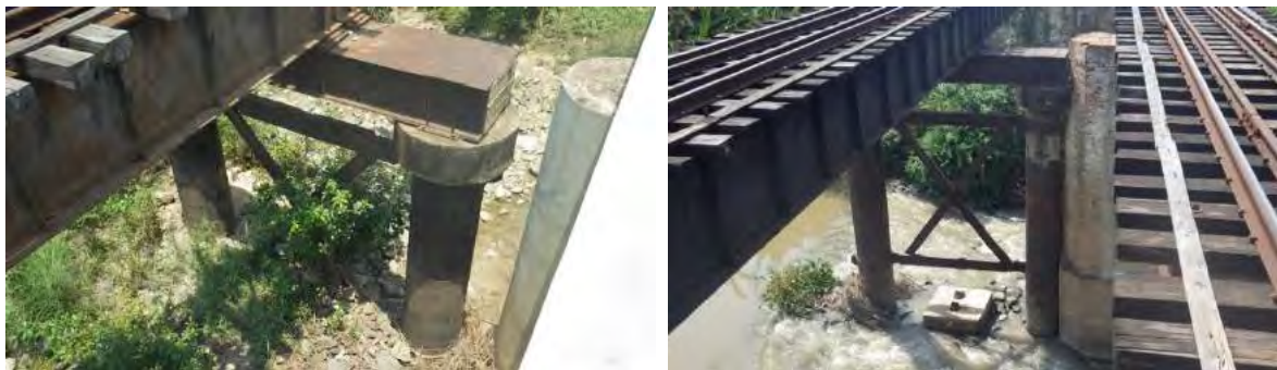
(a) Bridge No.727
