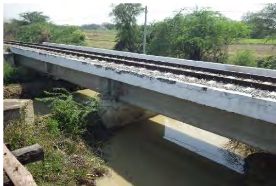
Prestressed Concrete Girder
