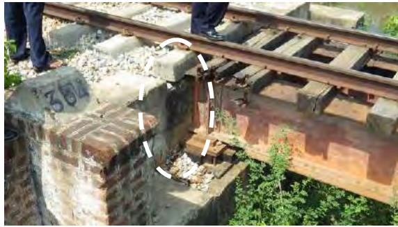
(a) Bridge No.384
