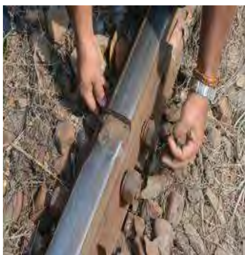
Figure 5.3.3 Damage at rail head
