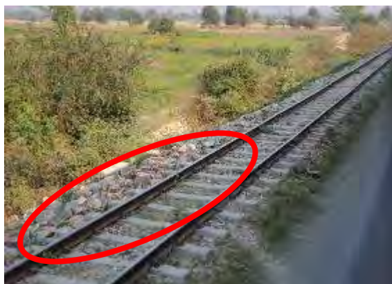
Figure 5.3.2 Distribution of Extremely Big Size Ballast Stones
