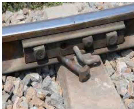
Figure 5.3.4 Missing of Rail Fish Bolts
