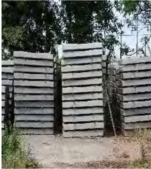
Figure 5.3.37 Stored PC Sleepers
