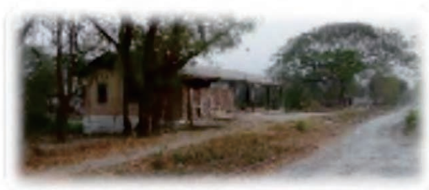
(Current Condition: Railway Track and Station)
