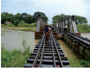
Photo.1 Water Condition under bridge (Mile 83)
