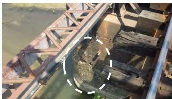
(b) Bridge No.306
