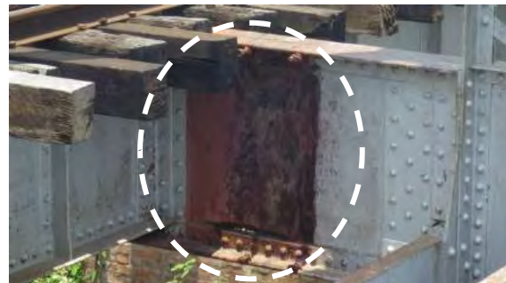
(b) Bridge No.730
