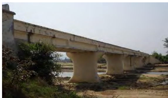
(a) Bridge No.453
