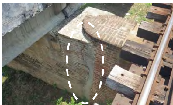
(c) Bridge No.519
