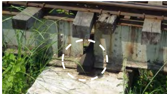
(c) Bridge No.320A
