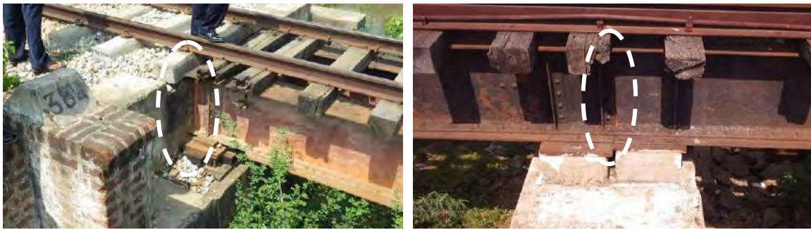
(a) Bridge No.384
