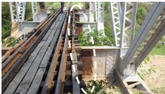
(a) Bridge No.453
