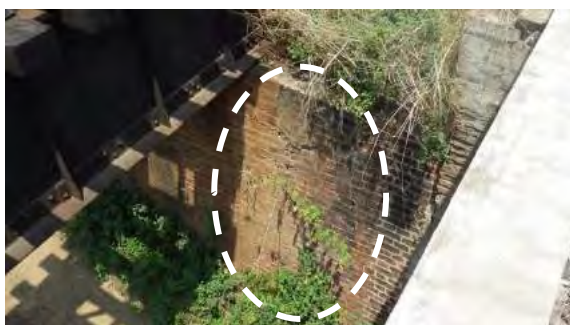
(a) Bridge No.497
