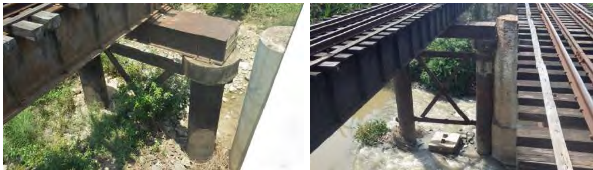
(a) Bridge No.727
