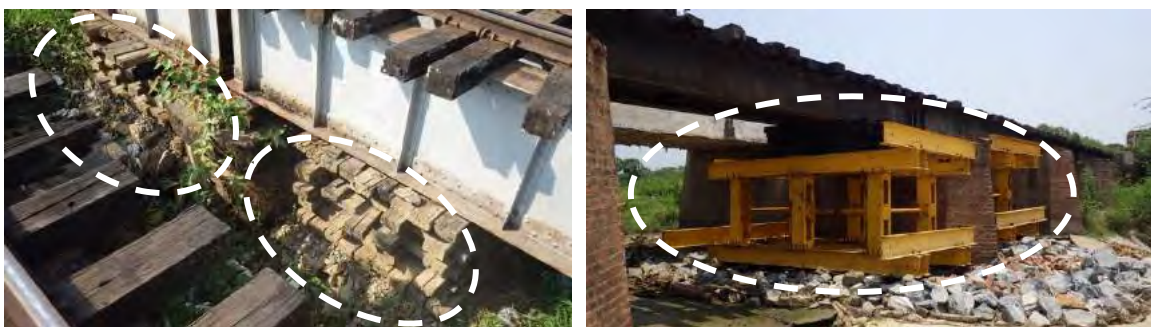
(a) Bridge No.270
