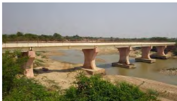
(b) Bridge No.691
