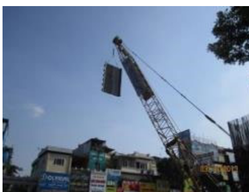
Figure 6.2.12 Trespassing on the Road by Lifting Objects (Hanoi Urban Railway Project)
