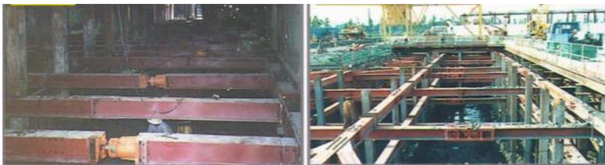
Figure 6.1.1 Propping with Pre-loading Method
