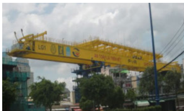
Figure 6.1.8 PC-U Segment Girder Installation by Steel Box Girder Gantry (HCM Line 1)
