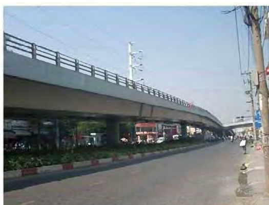
Figure 6.1.2 Cay Go Flyover
