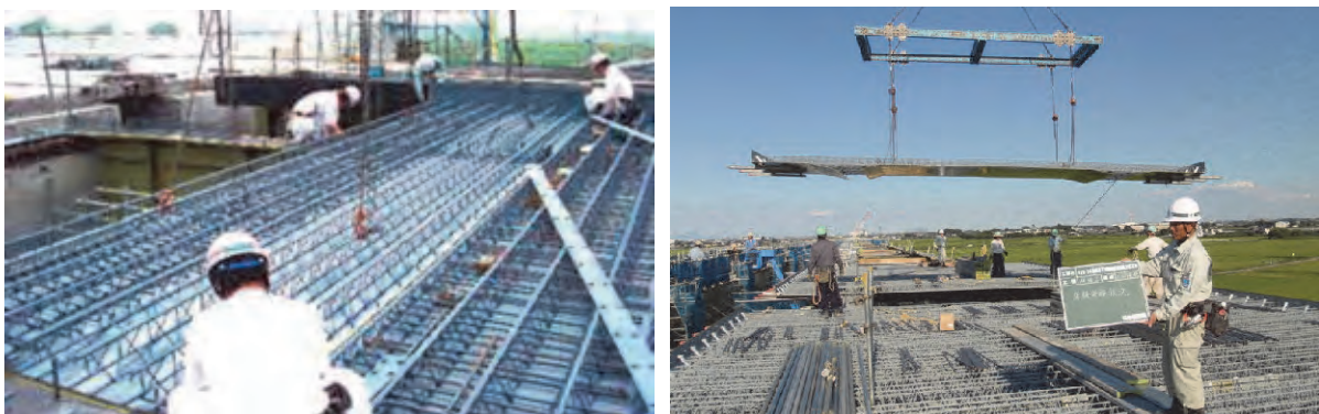
Figure 6.2.14 Example of Construction Works of Composite Slab
