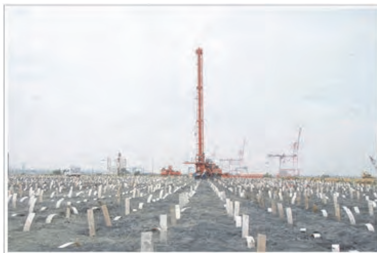
Figure 6.2.3 An Example of Plastic Board Drain Method
