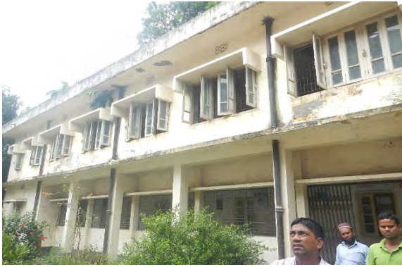
Shaturia Upazila Health Complex (UHC)
