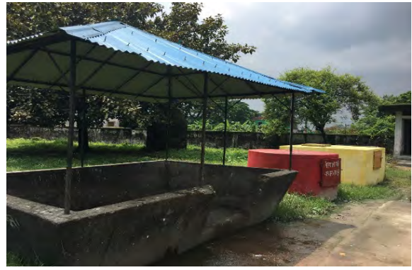
Solid waste facility, Narsingdi 100 bed District Hospital
