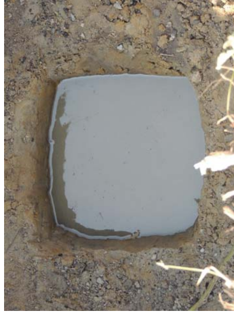
Figure 14. Pre-soaking the hole
