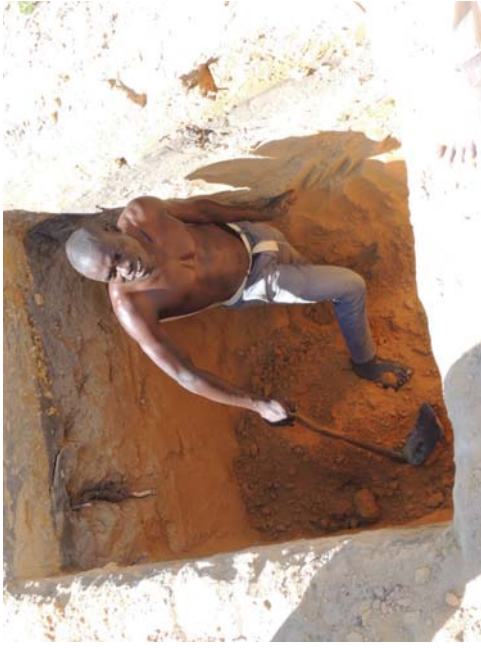
Figure 11. Excavation of Trial Pit, sampling at 1.75m
