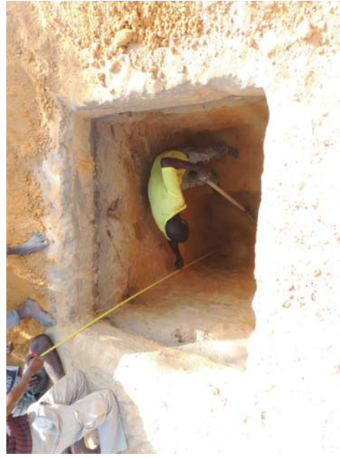
Figure 12. Excavation of Trial Pit, sampling at 2.5m
