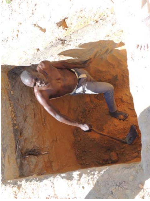
Figure 11. Excavation of Trial Pit, sampling at 1.75m
