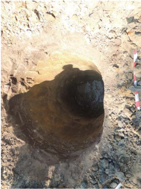
Figure 11. Excavation of Trial Pit, sampling at 1.75m
