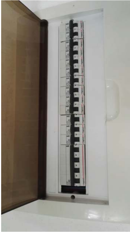
Figure 22. EB at the Administration Building
