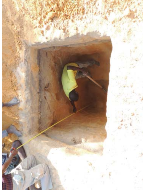
Figure 12. Excavation of Trial Pit, sampling at 2.5m
