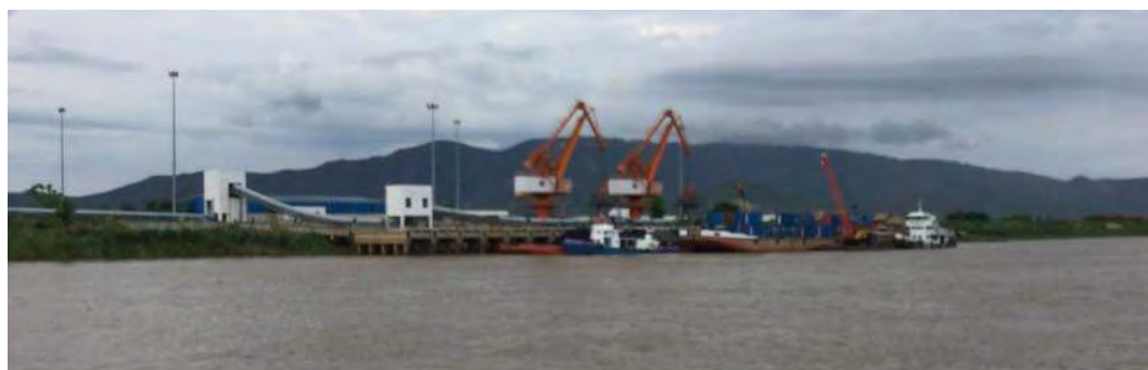
Photo 1-2-24 Fixed Jetty Structure near Takaung Town
