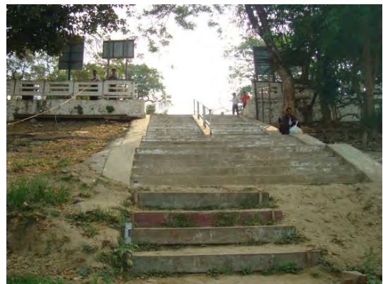
Photo 1-2-9 Access Step to Pontoon
