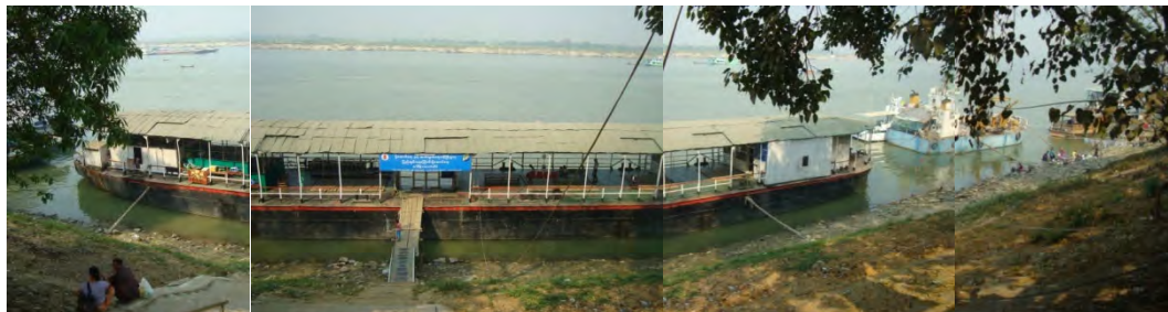
Photo 1-2-7 Passenger Terminal for IWT Operated Ships (Pontoon)
