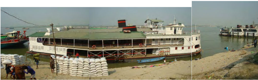
Photo 1-2-2 Ship Berthing Conditions along the Natural Riverbank
