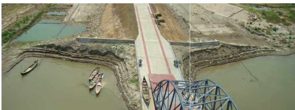
Photo 1-2-23 Sand Protection Wall
