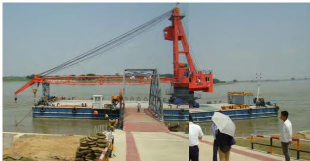
Photo 1-2-19 Semeikhon Port Pontoon
