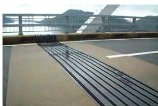
Figure 4.3.92 Sample of Modular Expansion Joint
