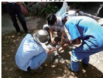
Installation of water level meter
