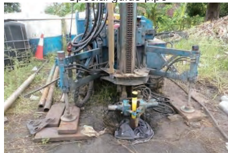
Setting of the guide pipe completed
