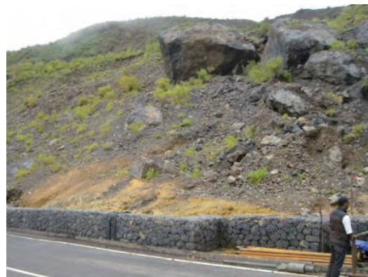
Figure 4.1.4 Gabion wall for Counter Weight (source: JET)
