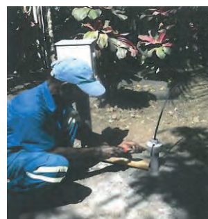
Installation of PVC pipe completed
