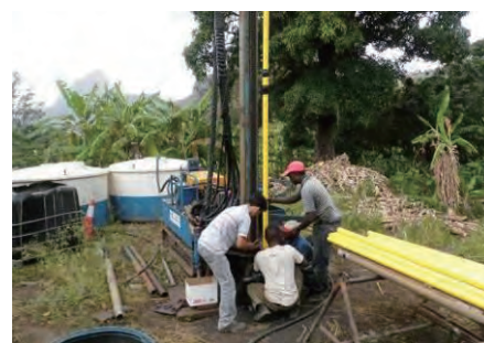
Insertion of the guide pipe
