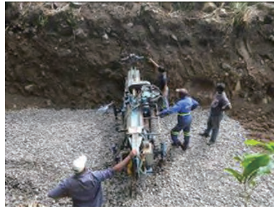
Photo A-2 Adjustment of drilling direction (Source: JET)
