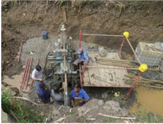
Photo A-4 Checking the inclination of drilling rod (Source: JET)
