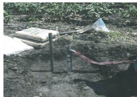
Setting of the pipe strain gauge complete
