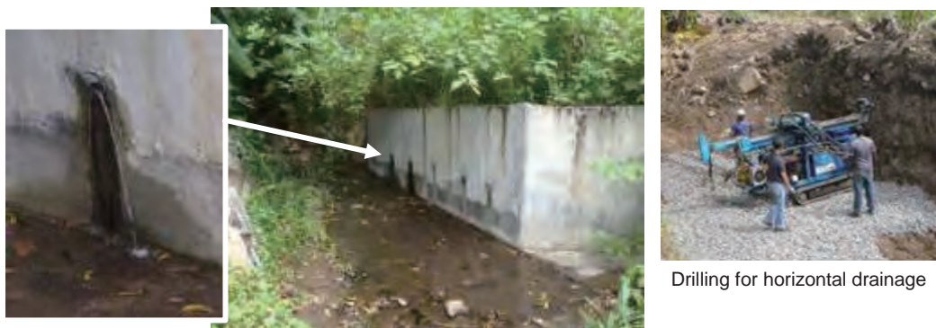
Figure 6.2.8 Horizontal Drainage, Chitrakoot (source: MPI)
