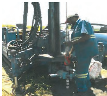
Installation of the pipe strain gauge
