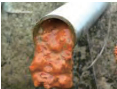
Photo 7.5.1 Slime in the Drainage Pipe 3
