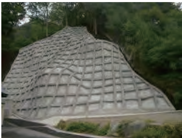
Figure 3.13 Example of Spray Crib works (source: JET)
