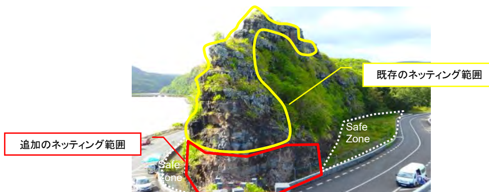
Figure 7 All of the tip of the cape should be covered with a lock net, Maconde
