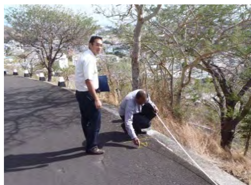
Photo 3 Drawing additional distance signs on the road (Source: JET)
