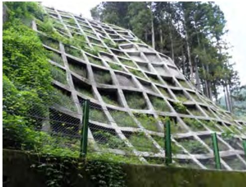
Photo 10 An example of a crib wall in Japan (Source: JET)
