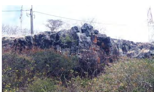
Photo 9 Planned location for a rockfall protection net at the top of the hill (Source: JET)
