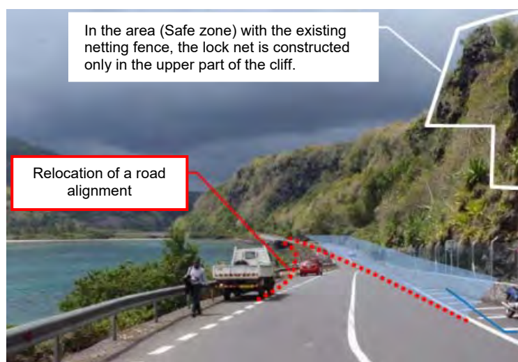
Figure 8 Relocation of a road alignment
