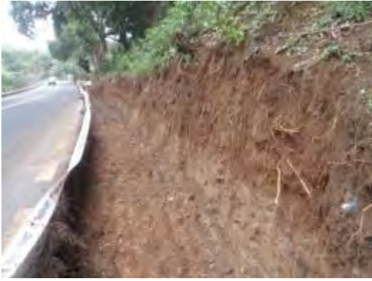
Excavation for the foundations
