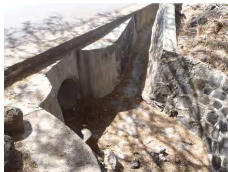
Photo 7 An example of an intact drainage (Source: JET)
