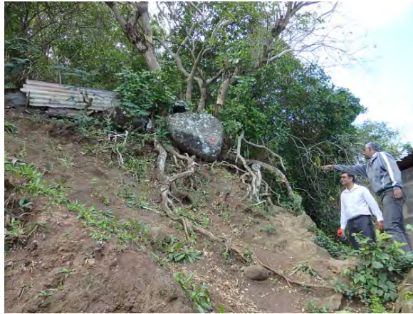
Photo 20 Consideration of measures (red spray: removal) (Source: JET)
