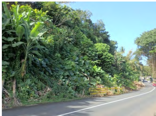
Photo 3 The slope at middle of the road in which a crib wall is to be applied (Source: JET)
