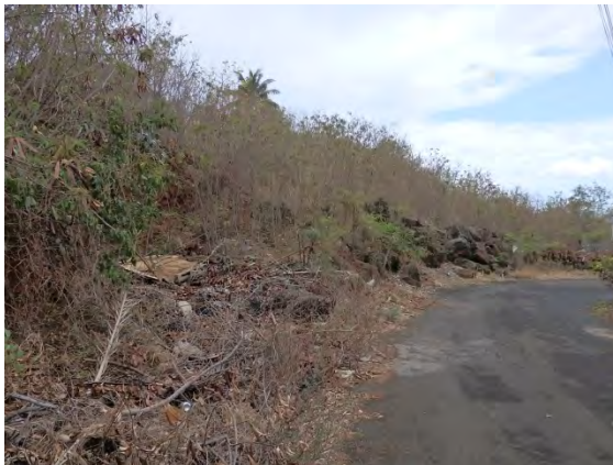
Photo15 A view of the slope (Source: JET)
