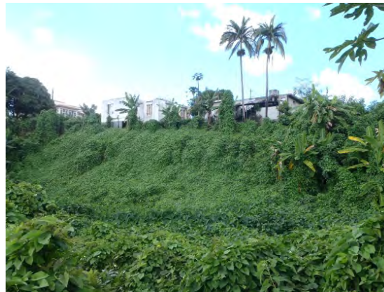
Photo 21 The investigation spot. Two houses sit near the scarp (Source: JET)
