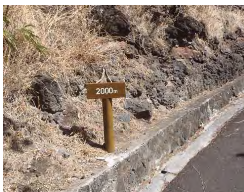
Photo 2 Existing chainage (Source: JET)
