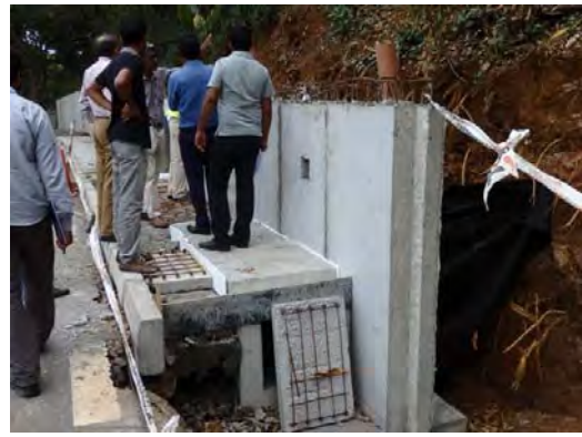
Completed retaining wall at a place of possible slope failures
