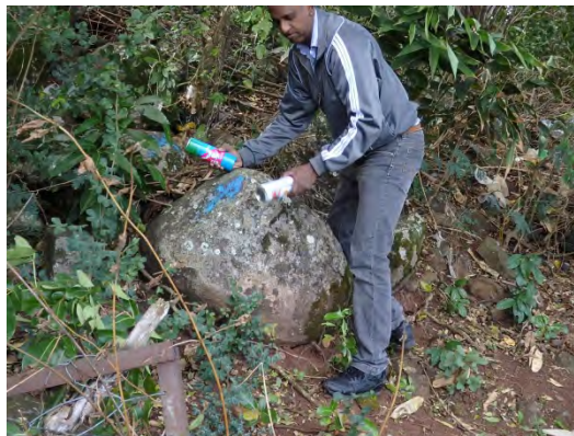
Photo 19 Consideration of measures (blue spray: stabilisation) (Source: JET)
