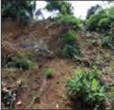
Slope Collapsed from the Top
