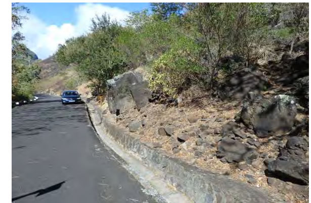
Photo-3 Slightly cut slope. Many unstable rocks can be seen. No barrier exists on the slope to the road.
