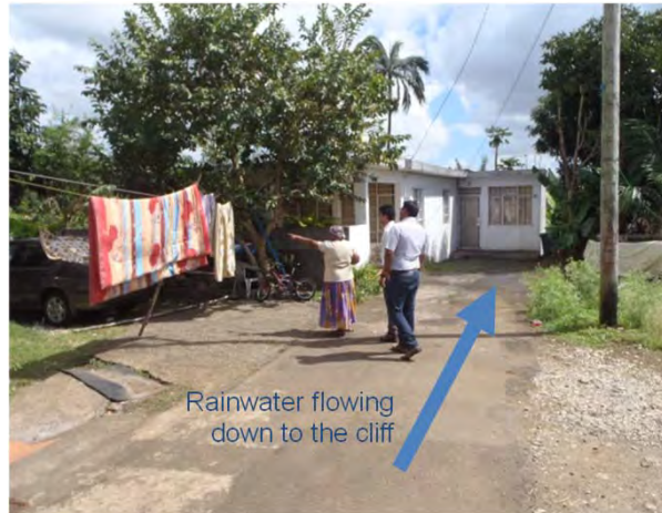
Rainwater flowing down the cliff from the road accelerates erosion of the cliff.
