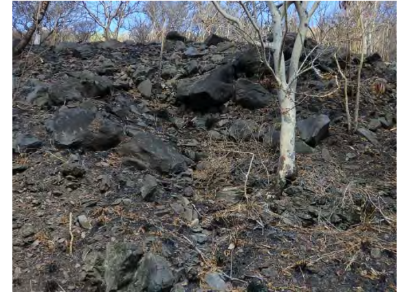
Photo-3 Slightly cut slope. Many unstable rocks can be seen. No barrier exists on the slope to the road.
