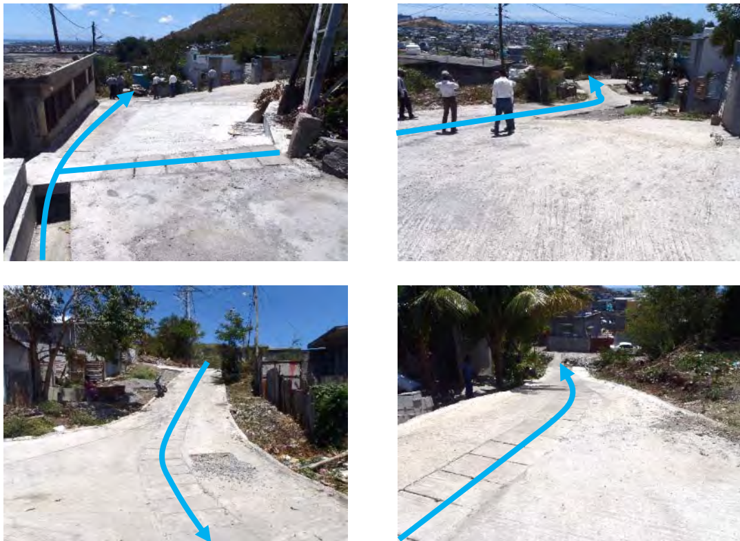
Figure 2 Surface drainage system in Valle Pitot, 12 th Oct 2017 (Source: JET)
