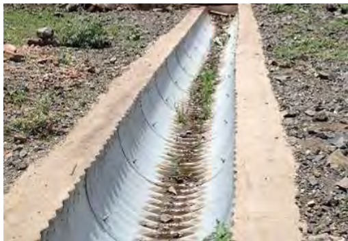
Restoration using corrugated pipe
