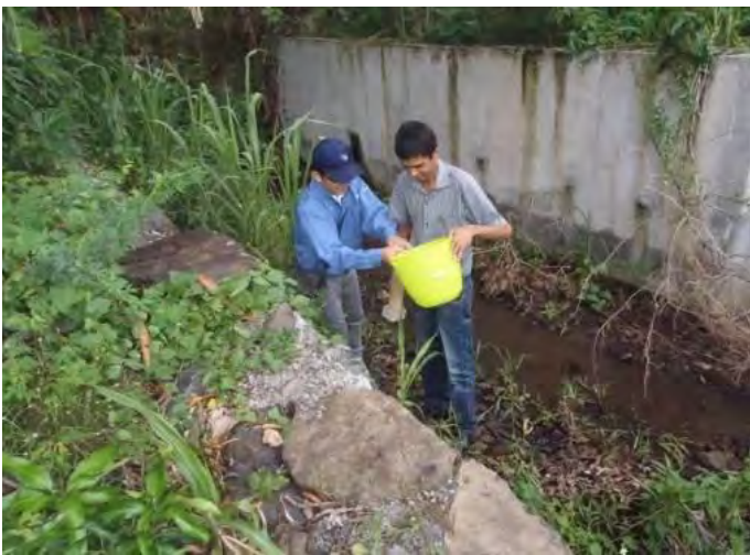
Measuring at the horizontal drainage constructed under the Previous Project, Chitrakoot
