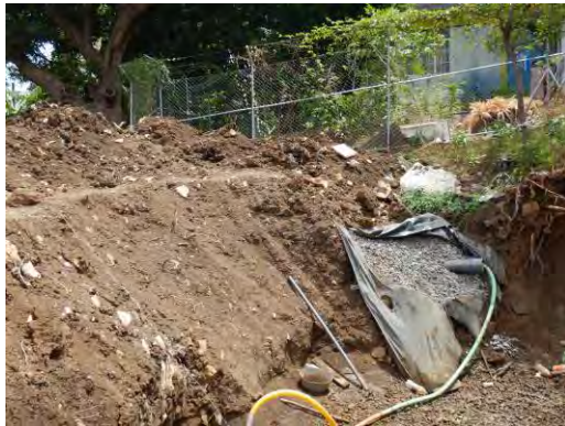
A1: Blind Ditch (Source: JET)
