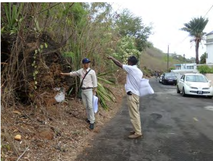
Site study of slope failure and rockfall, Hermitage
