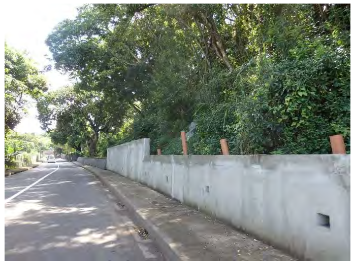
Completed countermeasure work, Batelage
