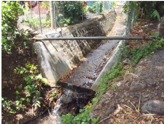
Photo 3 End part of the Reinforced Upgrade Drainage, RUD-1, March 2017
