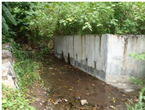
Photo 3 View of landslide countermeasure, horizontal drainage, HD-1, 08 th March 2016 (Source: JET)
