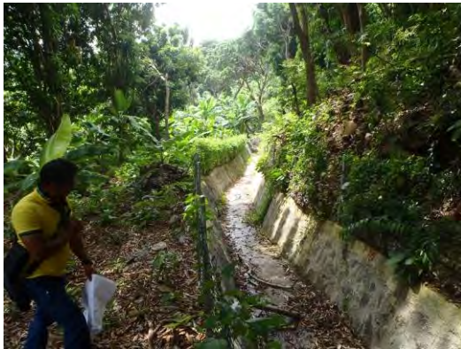
Photo 1 View of landslide Countermeasure, channel for flood, CH-1, 08 th March 2016 (Source: JET)
