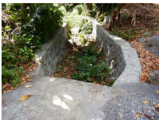
D.1: Upgrading of Existing Affluent
