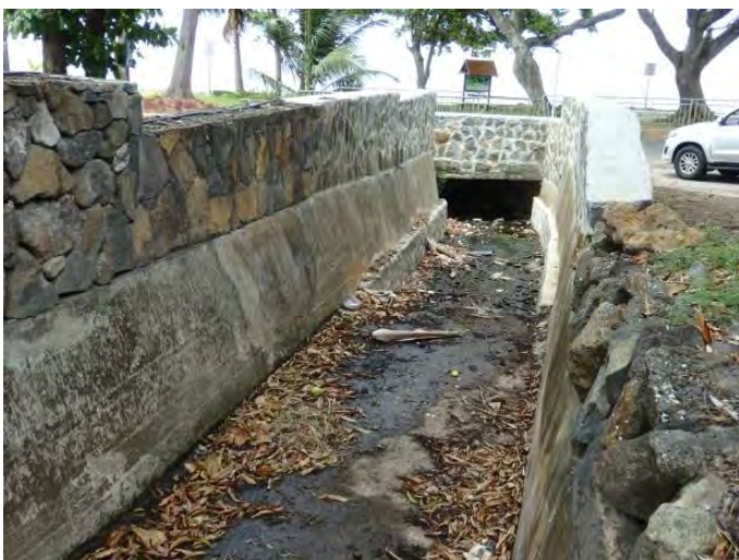
Countermeasure work for debris flow, Baie du Cap
