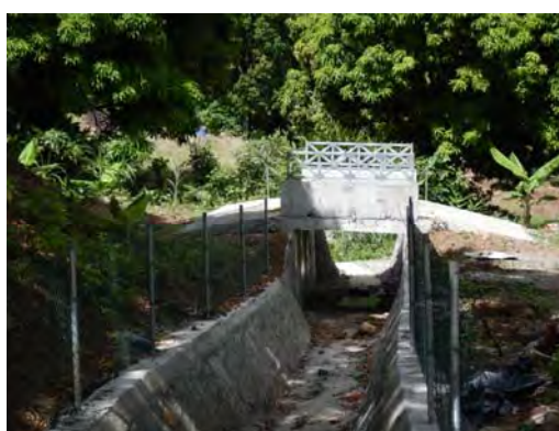
D.3: New Bridge NB1
