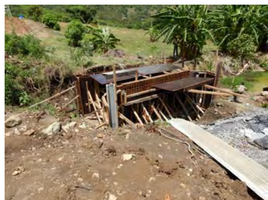
A.8: Vehicular Bridge
