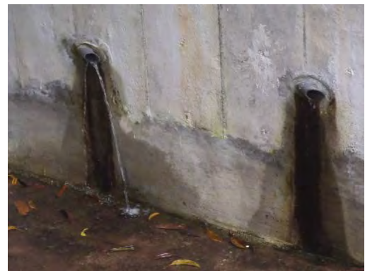
Photo 3 View of landslide countermeasure, horizontal drainage, HD-1, 08 th March 2016 (Source: JET)
