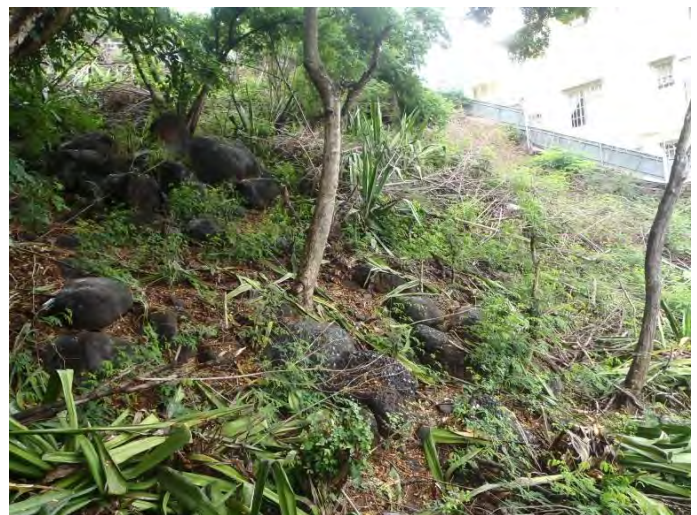
Unstable boulders on the steep slope, Coromandel
