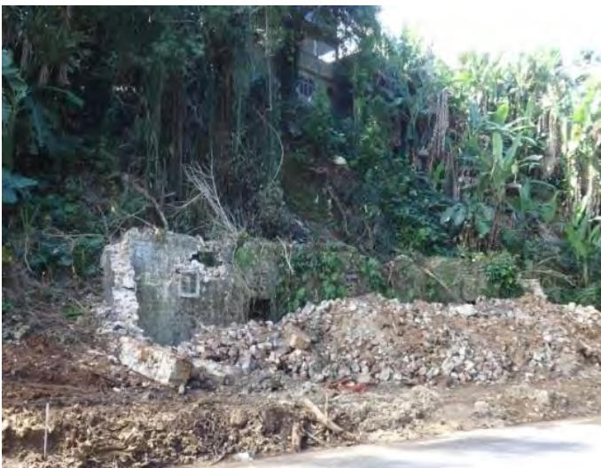
The slope in which a retaining wall (1.5 m high) is to be applied, Batelage
