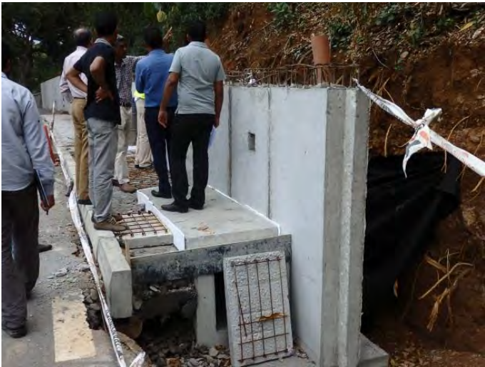
Construction of retaining wall at a place of possible slope failures, Batelage
