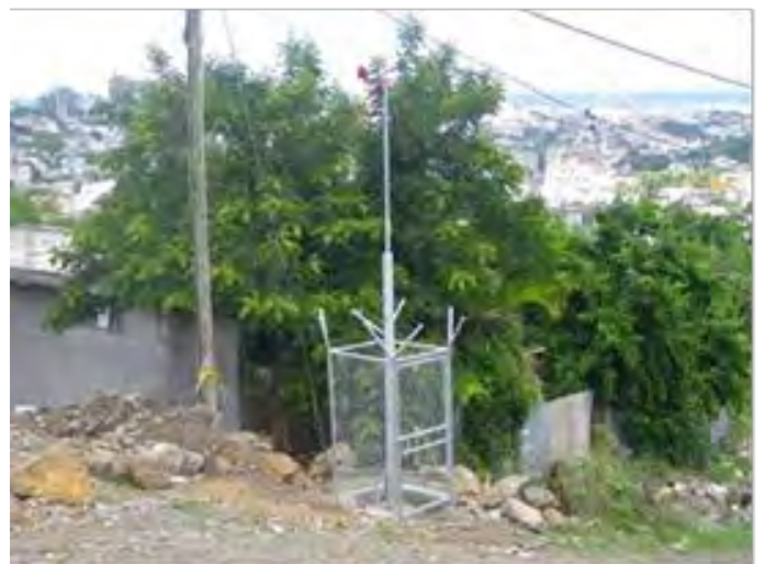
Early warning system, Vallée Pitot
