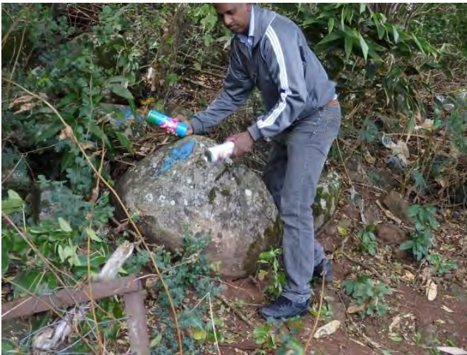
Consideration of measures (blue spray: stabilisation), Ruisseau Des Creoles
