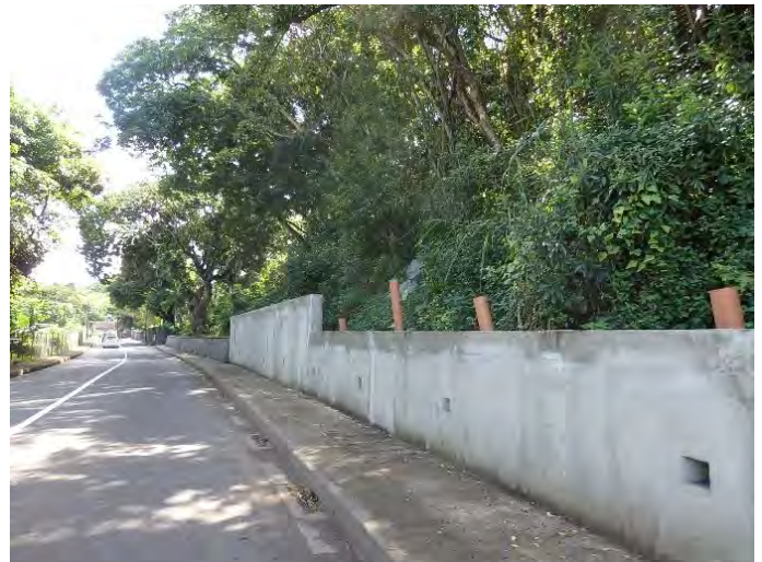
Completed countermeasure work, Batelage
