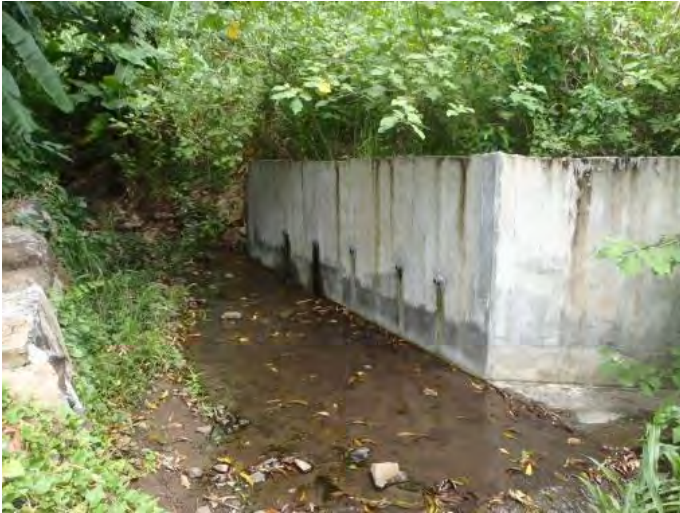
Landslide countermeasure constructed under the Previous JICA Project, Chitrakoot
