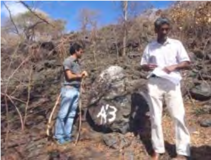
Specification of unstable rocks, evaluation, and numbering, Signal Mountain
