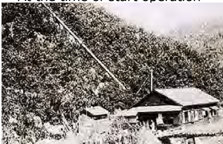
At the time of start operation
