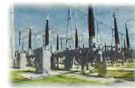
550kV Hybrid-GIS (H-GIS) China Southern Power Grid (China)
