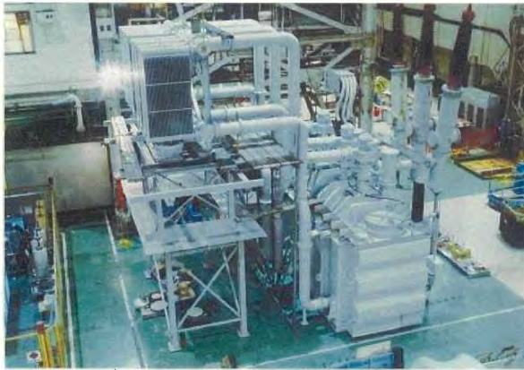
FOR UNDER GROUND SUBSTATION
