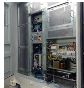
Battery Controllers
