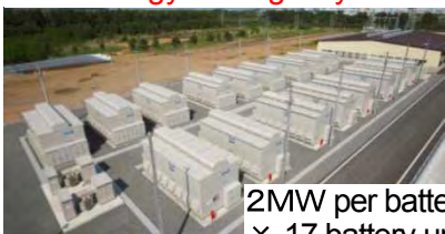
34MW (224MWh) NAS Energy Storage System
