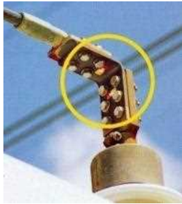
Checking overhead line termination
