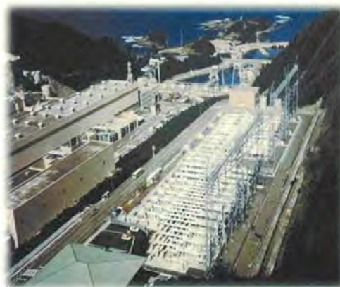
The world first 550kV Full-GIS Ohi Nuclear Power Plant (1976) Kansai Electric Power co. (Japan)
