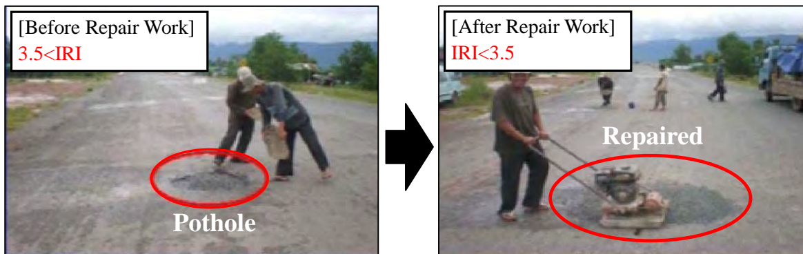
Figure-13 Comparison of Road Condition between before and after Repair Works
