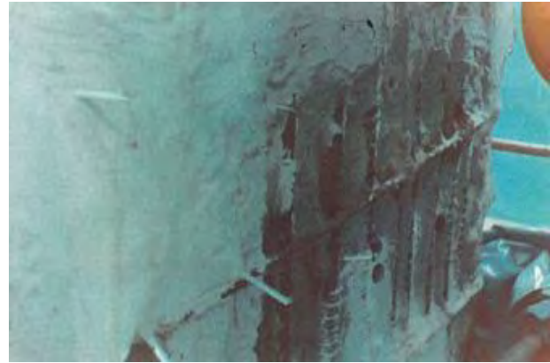
Photo 5.2.3.4 ជួសជុលដោយ putty sealant
