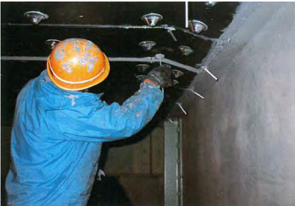
Photo 5.2.7.4 Attach steel plate
