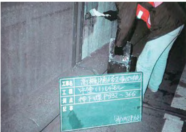
Photo 5.2.9.6 Tack-coating សំរាប់ intermediate coating
