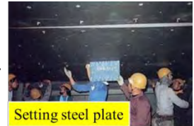
Setting steel plate
