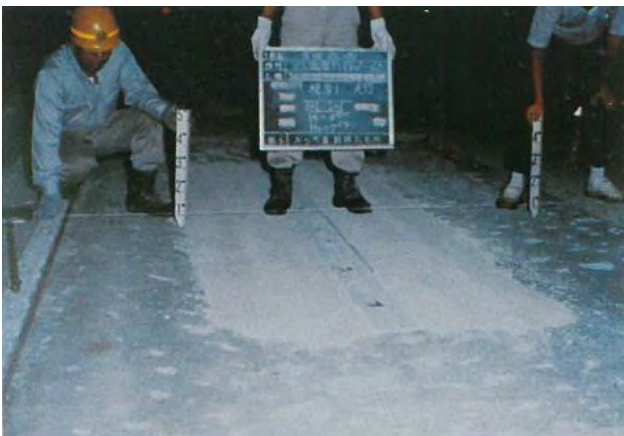
Photo 5.2.8.12 Checking re-concrete work
