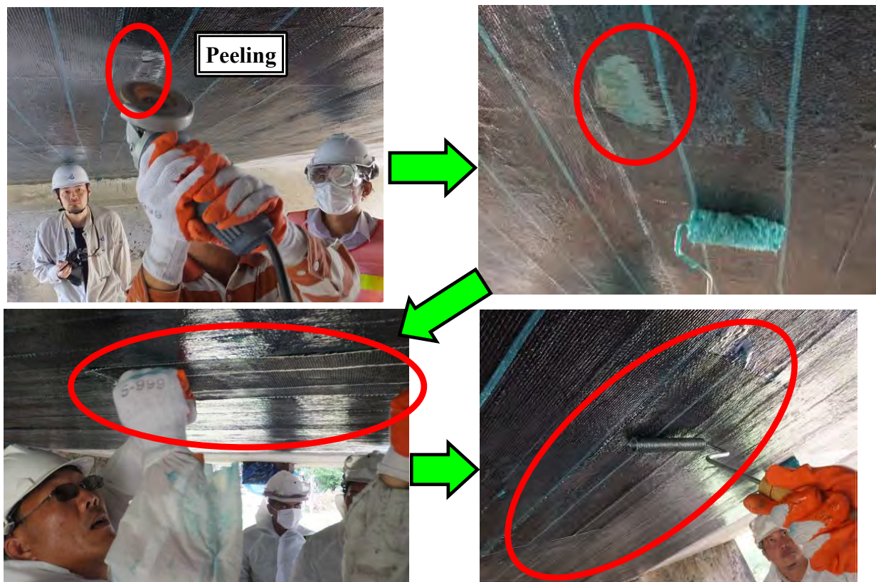
Photo 5.2.2.35 Repairing after completely cured impregnating resin
