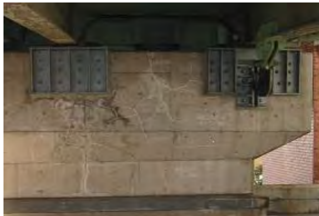
Photo 5.2.1.1 Concrete crack on pier
