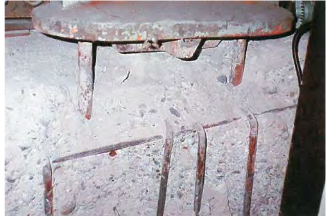
Photo 5.2.4.3 Damaged concrete chipped off
