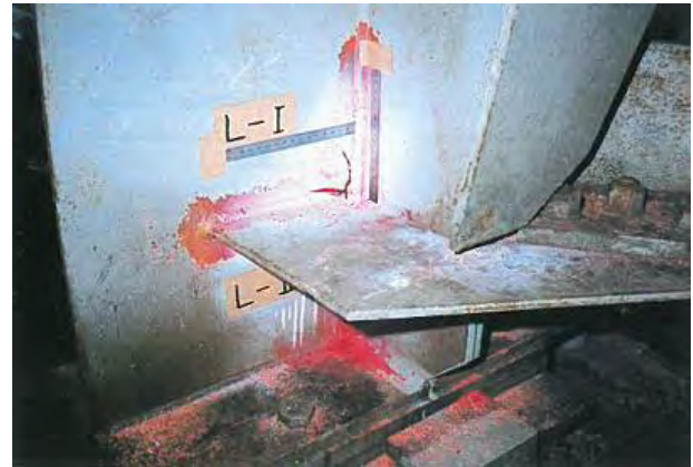
Photo 6.2.3.1 Condition of crack
