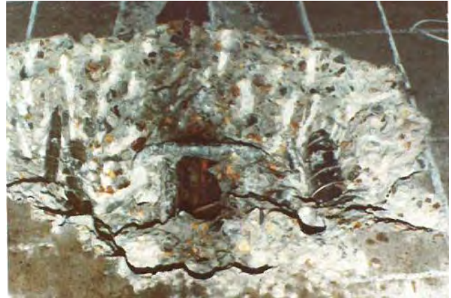
Photo 5.2.6.3 Lower flange after chipping-off
