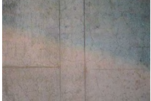
(b) B-5 panel damage
