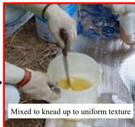
Photo 5.2.1.14 Mixing material (Epoxy resin material)
