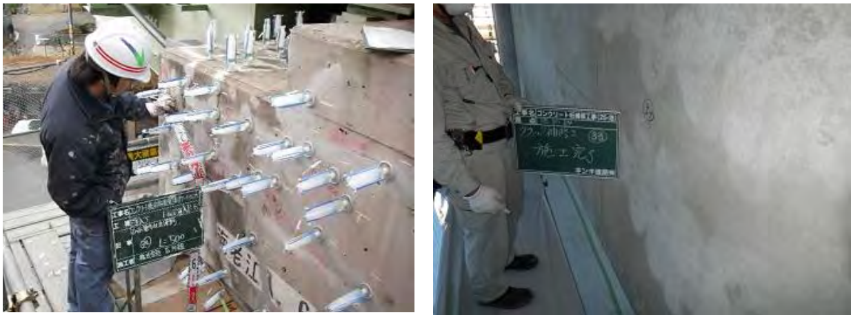
Photo 5.2.1.2 Concrete crack repair method
