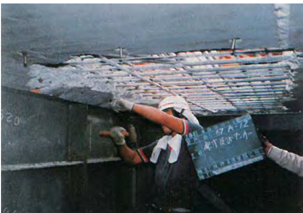
Photo 5.2.8.6 Driving of hole in anchor
