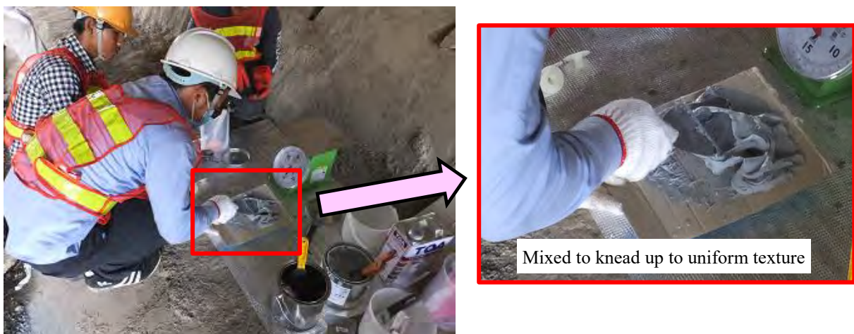
Photo 5.2.1.9 Mixing material (Sealing material)
