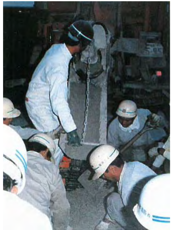
Photo 5.2.8.11 Placing concrete
