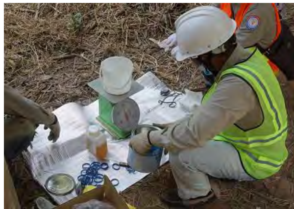
Photo 5.2.1.13 Weighing material (Epoxy resin material)
