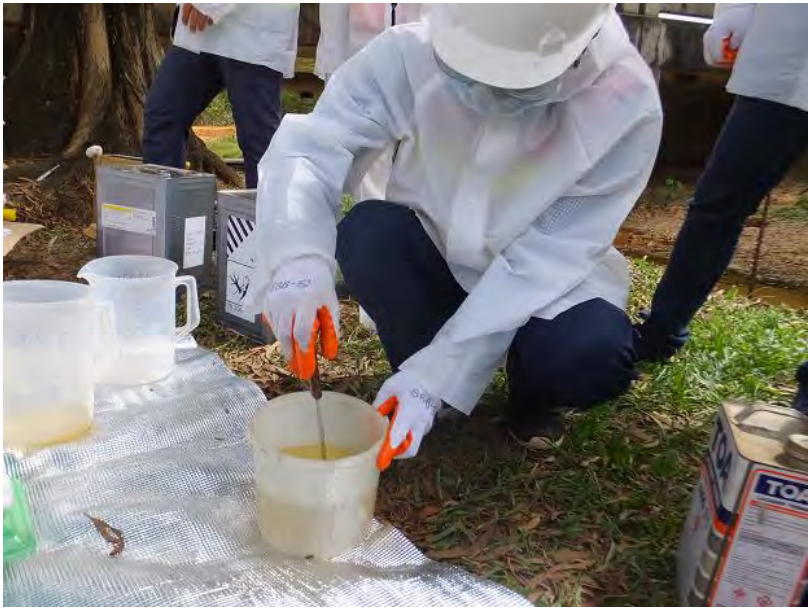
Photo 5.2.2.15 Mixing material (Primer material)
