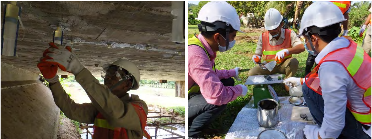
Photo 5.2.2.7 Crack repair (Reference: C-1 Concrete crack)
