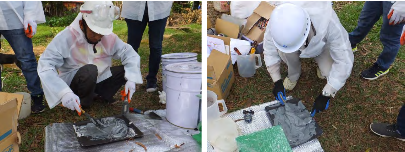
Photo 5.2.2.20 Mixing material (Smoothing agent material)
