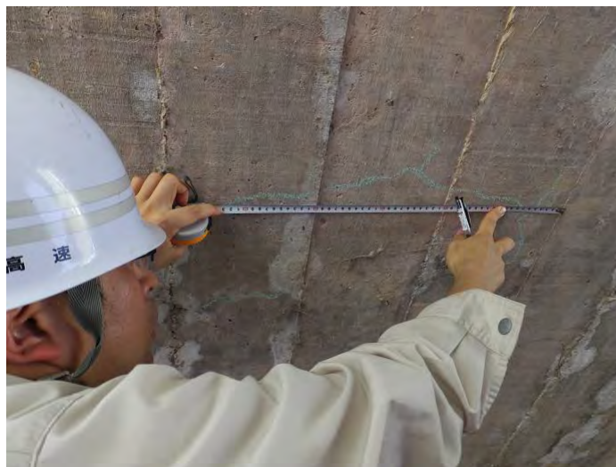
Photo 5.2.2.6 Measure the reinforcing range
