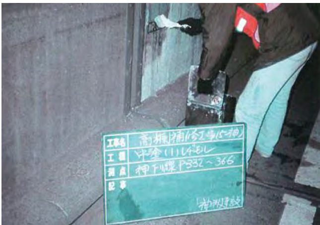
Photo 5.2.9.6 Tack-coating for intermediate coating
