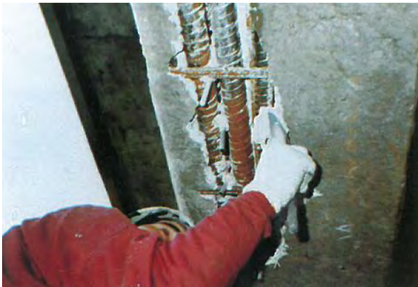
(a) Epoxy resin applied for the repair
