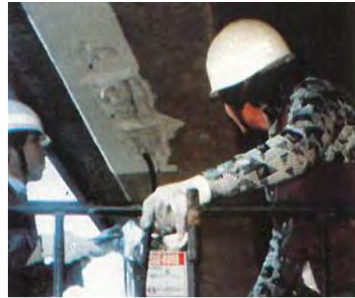
(b) Repair working
