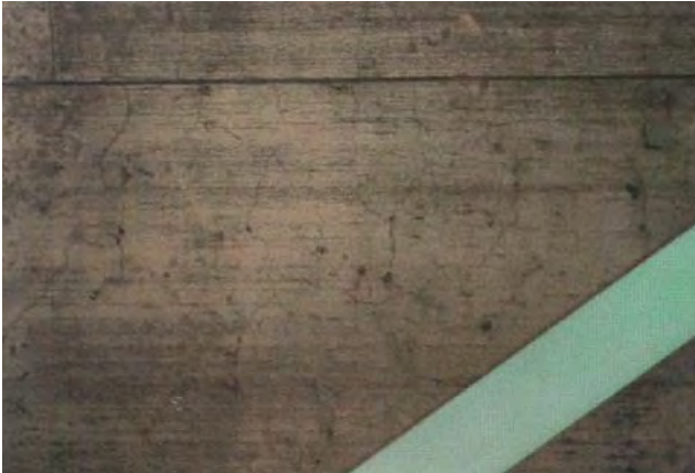
(a) A-4 panel damage
