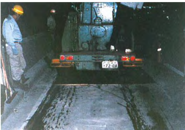
Photo 5.2.8.13 Pavement being placed and compacted
