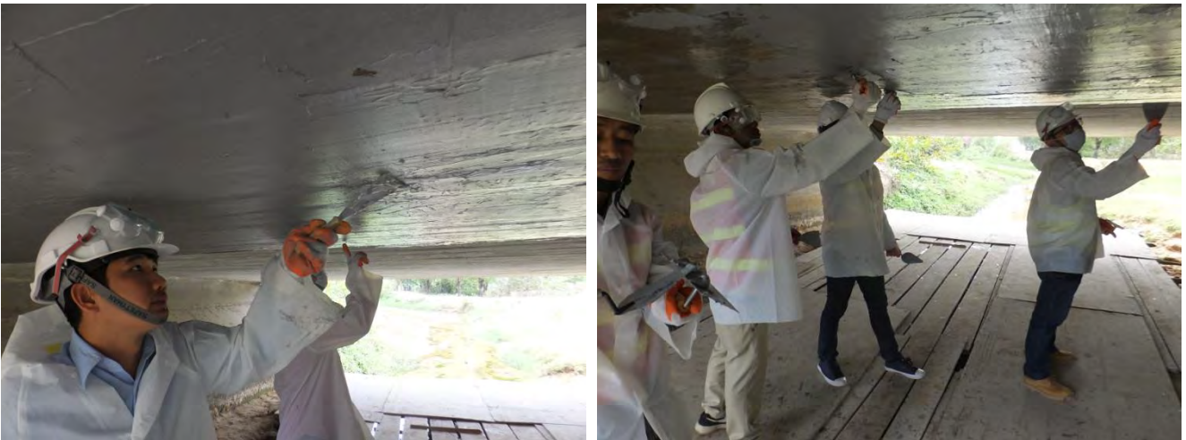
Photo 5.2.2.21 Applying smoothing agent
