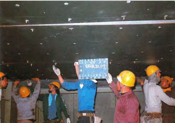
Photo 5.2.7.4 Attach steel plate
