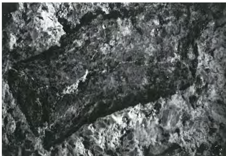
Photo 5.2.12.3 Reaction ring and crack inside of aggregate
