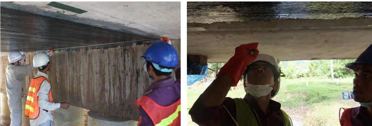
Photo 5.2.2.37 Measurement of CFC construction range
