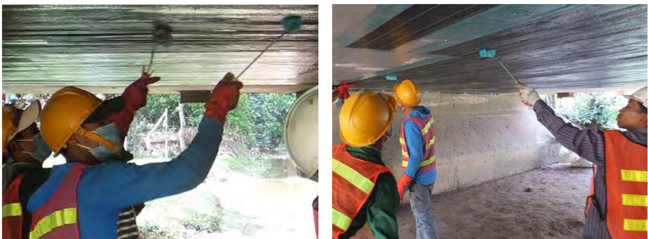
Photo 5.2.2.32 Applying 1st impregnating resin (once again)
