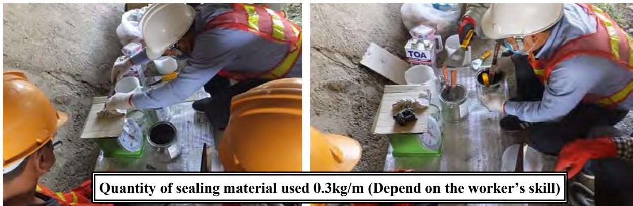
Photo 5.2.1.8 Weighing material (Sealing material)
