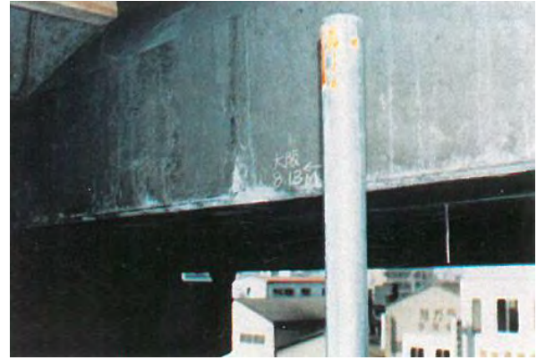
Photo 5.2.6.1 Deposit of free hanging like icicles
