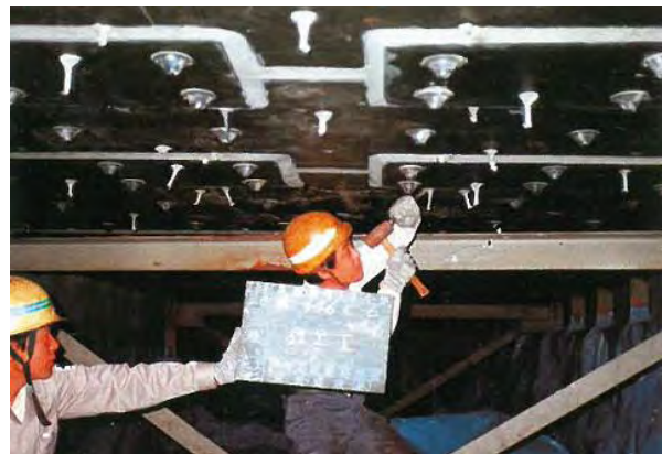
Photo 5.2.7.7 Cutting injection pipe
