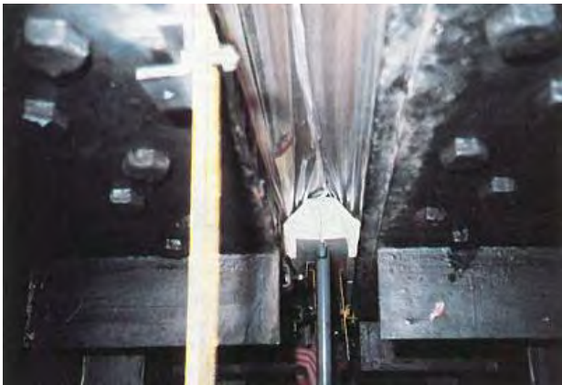
(a) Installation of back-up material
