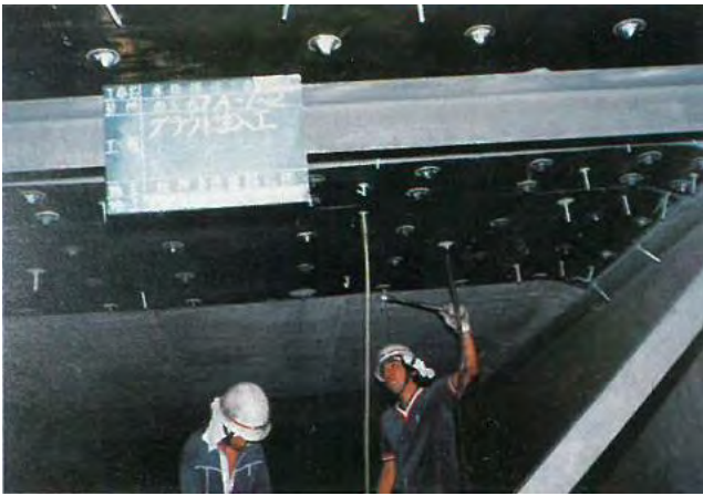
Photo 5.2.8.10 Resin injection
