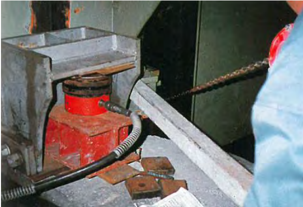
Photo 5.2.4.2 Temporary support by jack up
