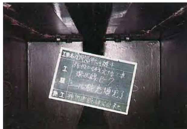
(c) Finished work
