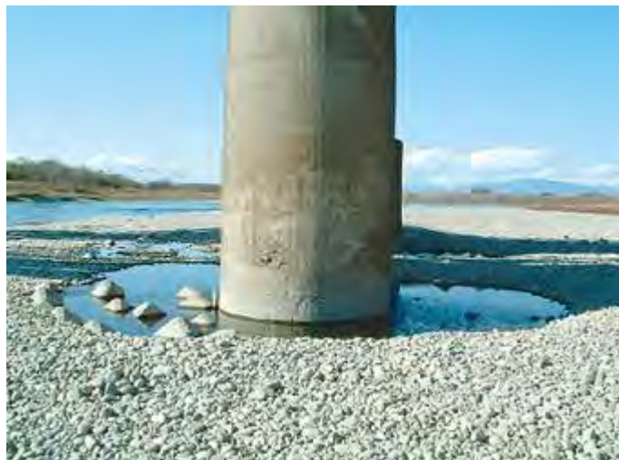
Photo 7.1.2.3 Schematic representation of scour at a cylindrical pier
