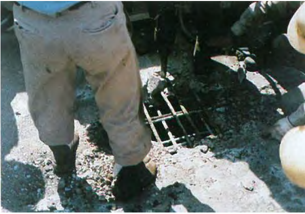
Photo 5.2.8.4 Slab concrete being chipped off
