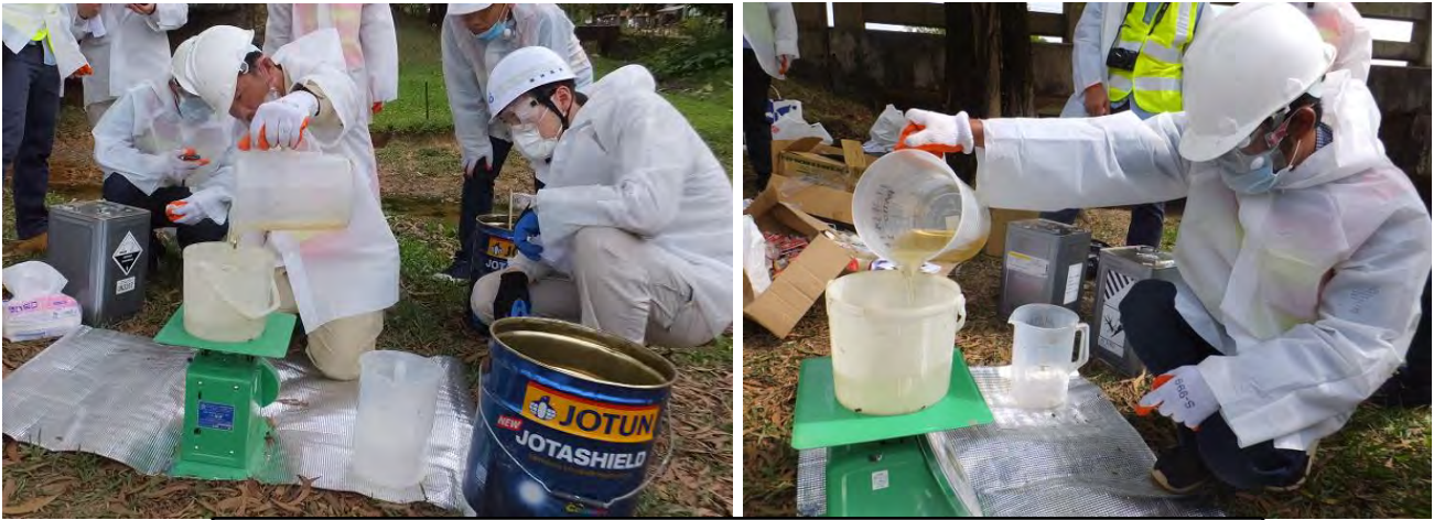
Quantity of primer material used 0.9kg/1 time (Main: Hardener = 0.6:0.3) 0.21kg/m 2 (Main: Hardener = 1.4:0.7) (Depend on the worker's skill)
