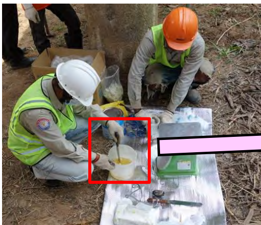
Photo 5.2.1.14 Mixing material (Epoxy resin material)
