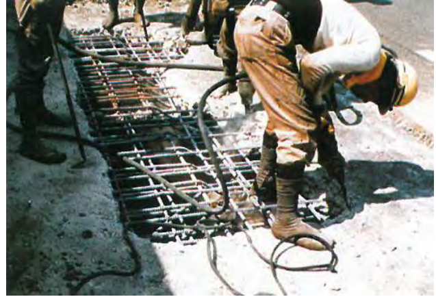
Photo 5.2.8.4 Slab concrete being chipped off
