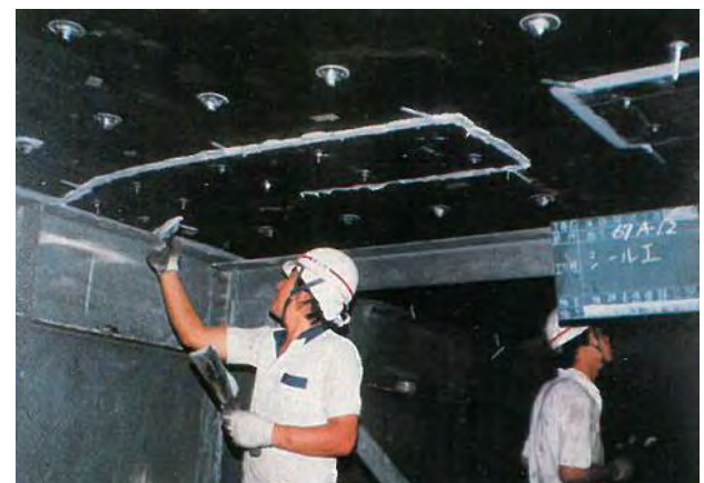
Photo 5.2.8.9 Injection pipes and sealing are installed
