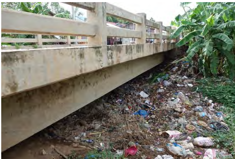
Photo 7.1.2.4 Trash under the bridge
