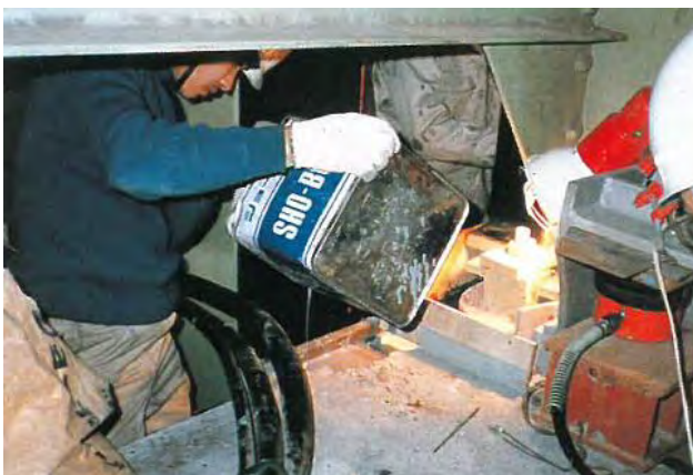
Photo 5.2.4.5 Poring epoxy resin
