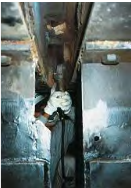
Photo 7.1.1.3 Cleaning of the web surface
