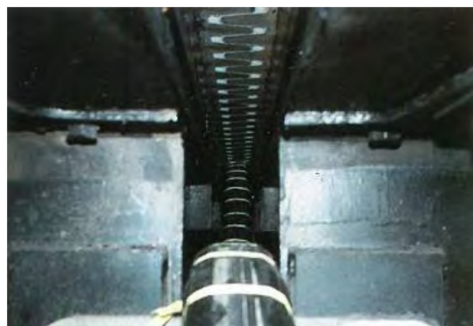
Photo 7.1.1.4 Setting of formed water cut-off material
