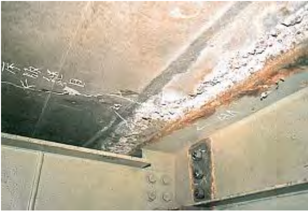
Photo 6.2.1.2 Water leakage from the construction joint of slab concrete
