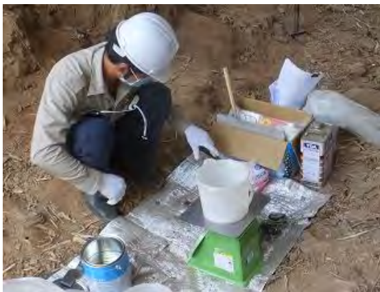
Photo 5.2.1.13 Weighing material (Epoxy resin material)
