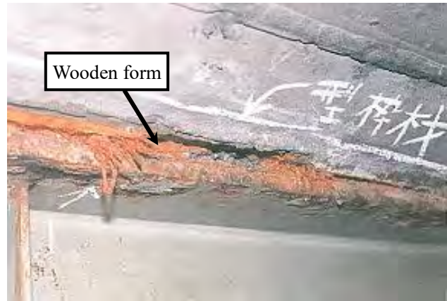
Photo 6.2.1.3 Wooden form which was left in the slab concrete
