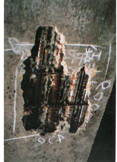
Photo 5.2.5.2 Condition after hammer-tapping
