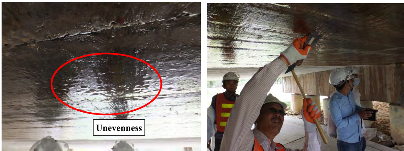
Photo 5.2.2.17 Confirmation of primer surface flatness
