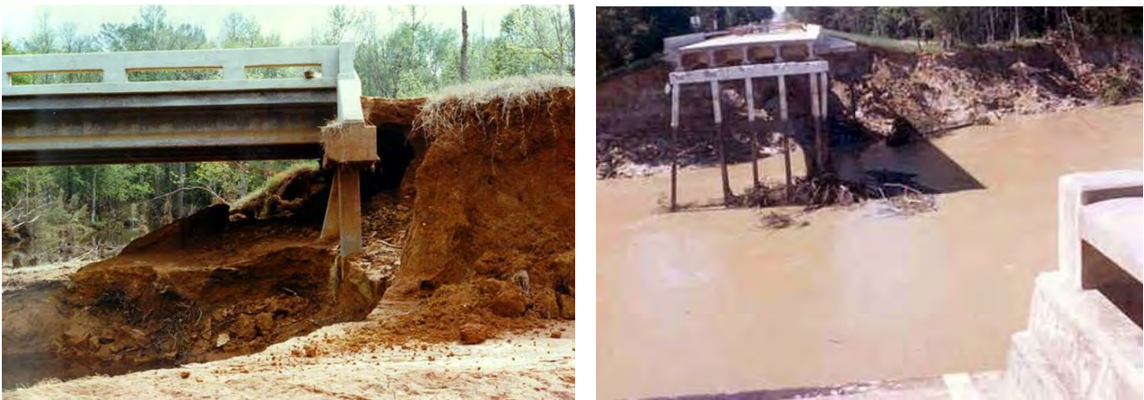
Photo 7.1.2.1 Condition of Bridge Score
