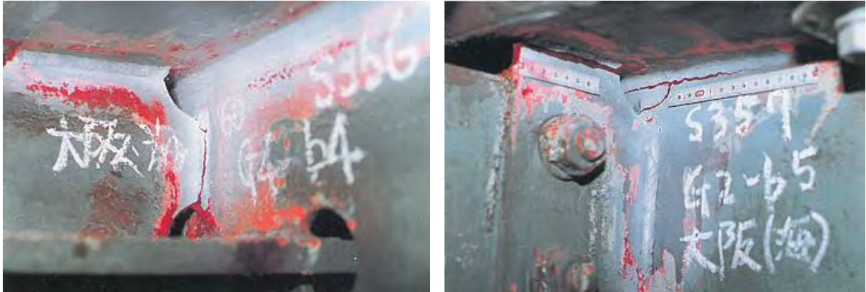
Photo 6.2.2.1 Cracks the jammed part connection cross beam and vertical stiffener of I-girder
