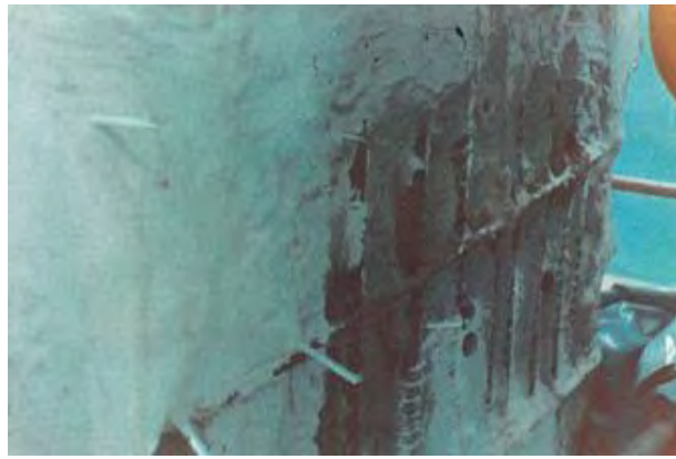
Photo 5.2.3.4 Repair by putty sealant
