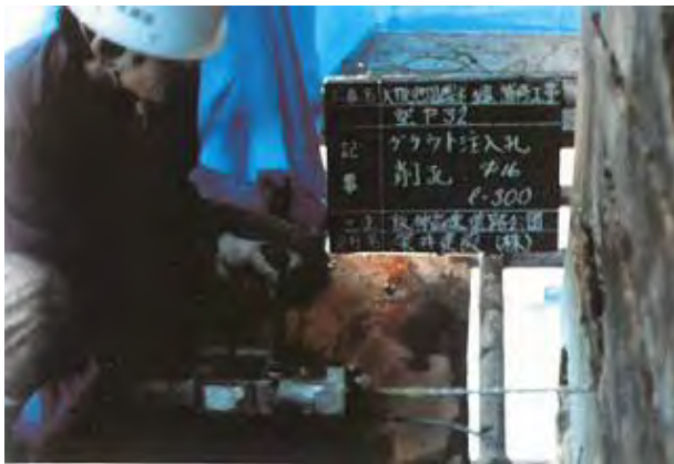
Photo 5.2.3.5 Grout injection hole provided
