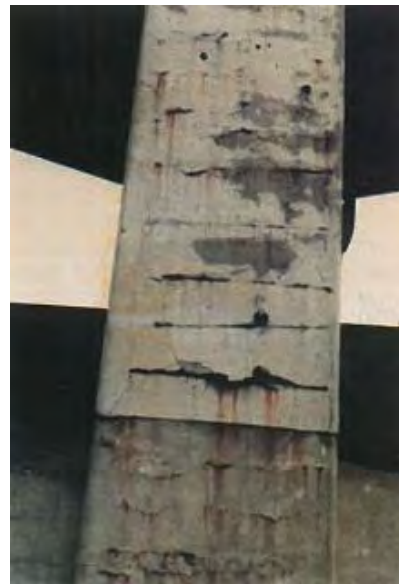
Photo 5.2.3.3 Exposed RE-bars and concrete flake-off
