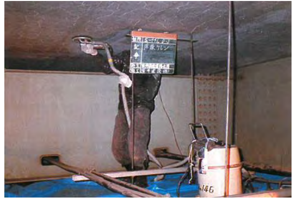
Photo 5.2.7.3 Cleaning of efflorescence on concrete surface
