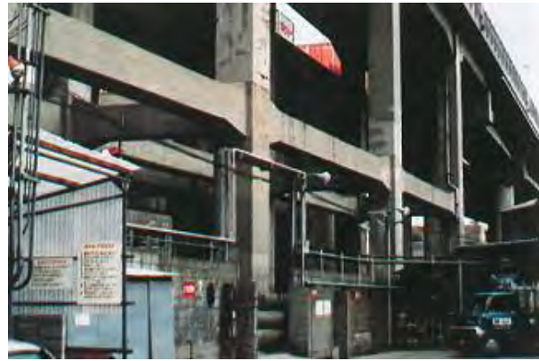
Photo 5.2.3.1 General view of damaged part
