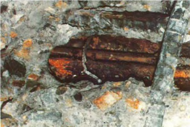
Photo 5.2.6.2 Steel wire exposed by hammering
