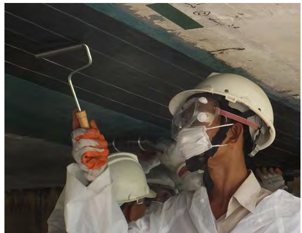
Photo 5.2.2.30 Pushing out air bubbles by paddle roller
