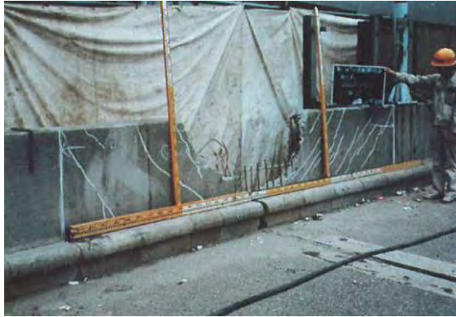
Photo 5.2.10.1 Damage condition (Case 1)
