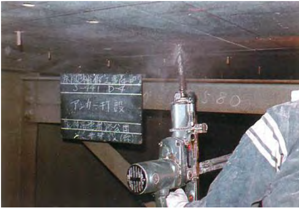
Photo 5.2.7.2 Driving of hole in anchor
