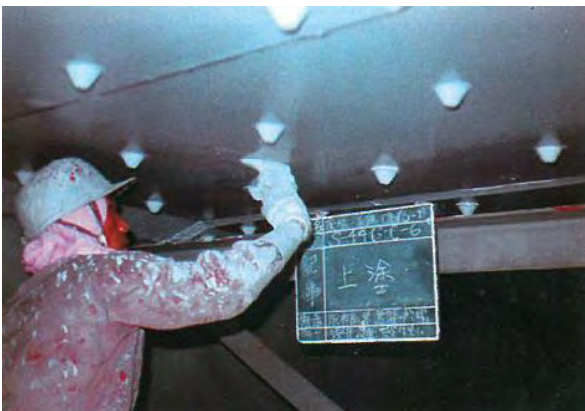
Photo 5.2.7.8 Painting of steel plate surface
