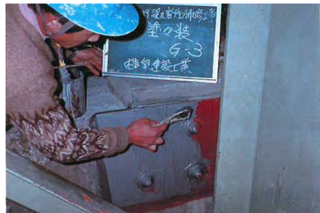
Photo 5.2.4.6 Reinforcing steel plate painted
