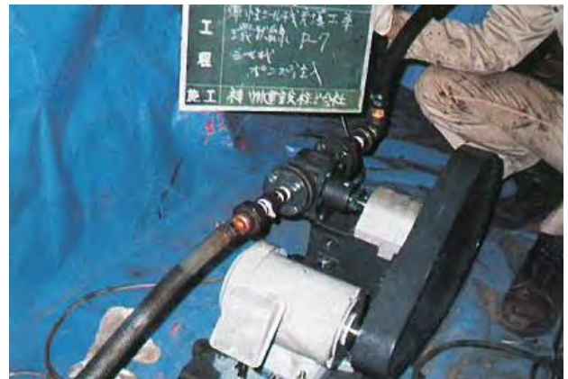
(b) Pouring of elastic sealing
