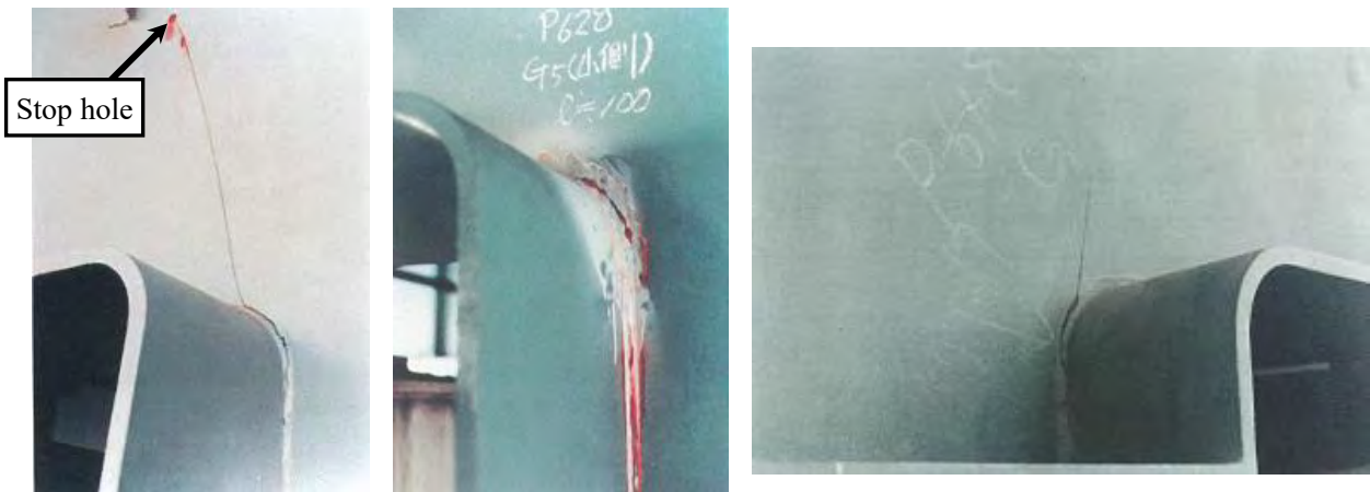
Photo 6.2.4.1 Crack on steel girder
