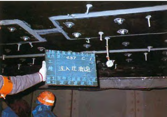
Photo 5.2.7.6 Measurement injection pressure
