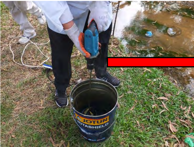
Photo 5.2.2.27 Mixing material (Impregnating resin)
