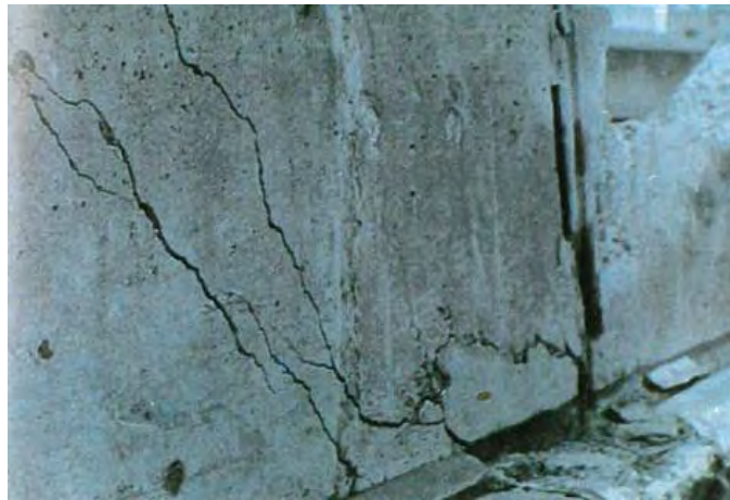
Photo 5.2.10.5 Damage railing (Case 3)
