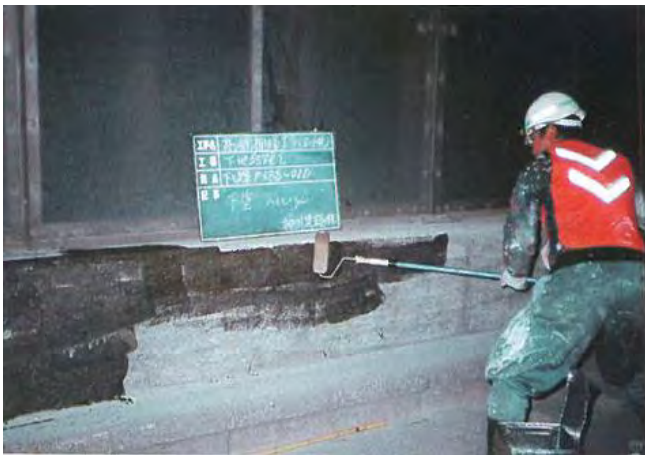
Photo 5.2.9.4 Primary coat painting
