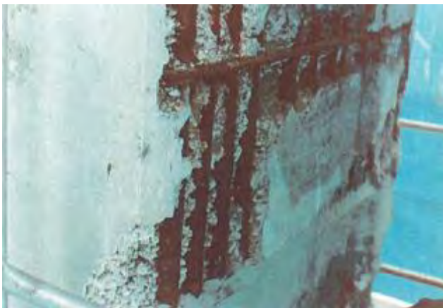
Photo 5.2.3.2 Concrete flake-off
