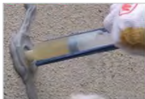
Injection into cracks with epoxy resin
