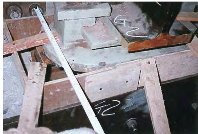
Photo 5.2.4.4 Steel plate being mounted
