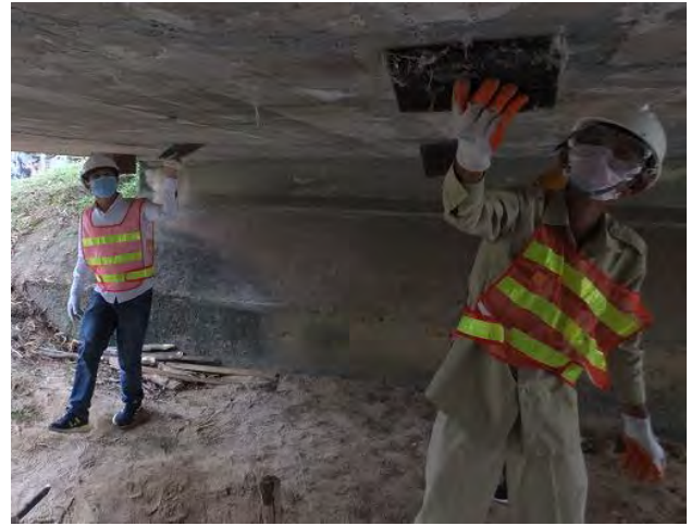
(b) To remove dust by polishing scrubbing
