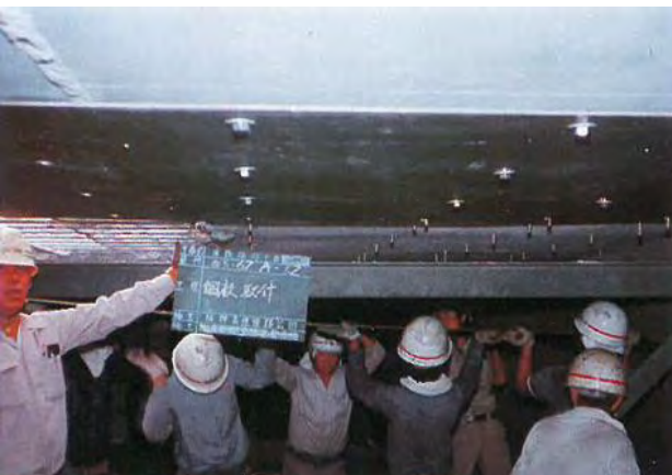
Photo 5.2.8.8 Steel plate attached
