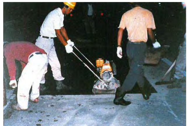
Photo 5.2.8.13 Pavement being placed and compacted
