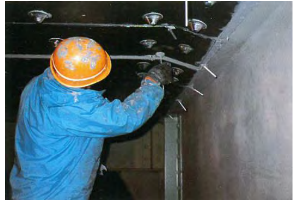
Photo 5.2.7.5 Sealing steel plate edge
