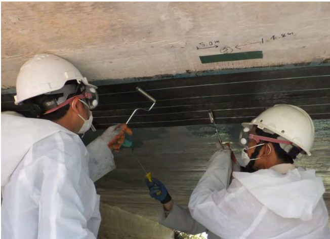
Photo 5.2.2.30 Pushing out air bubbles by paddle roller
