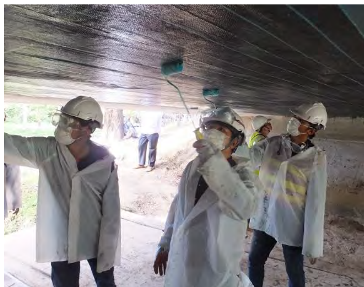
Photo 5.2.2.33 Applying 2nd impregnating resin
