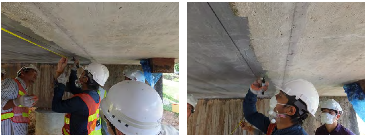
Photo 5.2.2.23 Measurement of CFC construction range
