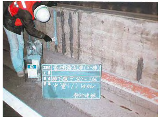
Photo 5.2.9.5 Tack-coating for second coat
