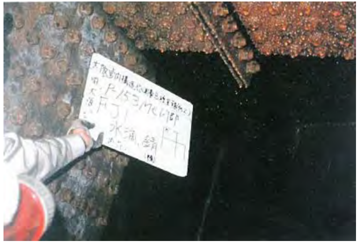
(b) Corrosion status (No painting)
