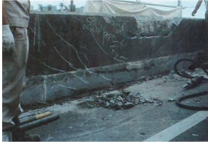
Photo 5.2.10.3 Damage condition (Case 2)
