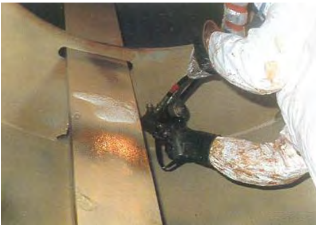
(c) Rigid urethane spraying
