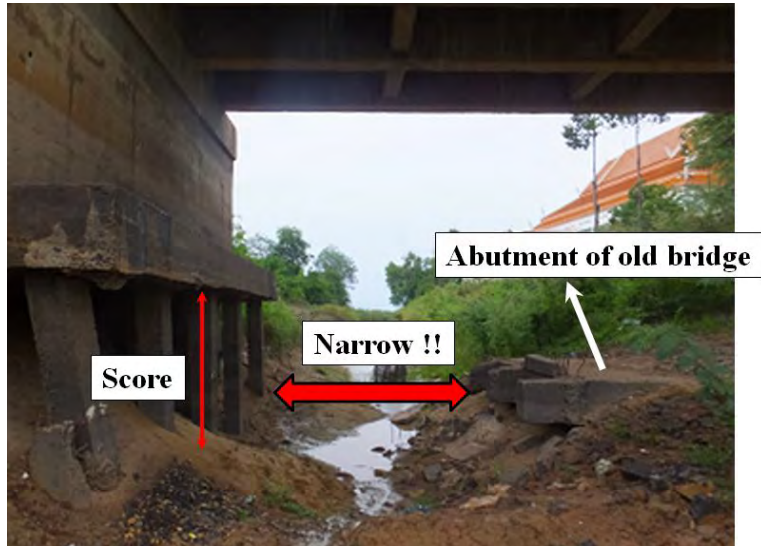
Photo 7.1.2.2 Narrow river width by old bridge abutment
