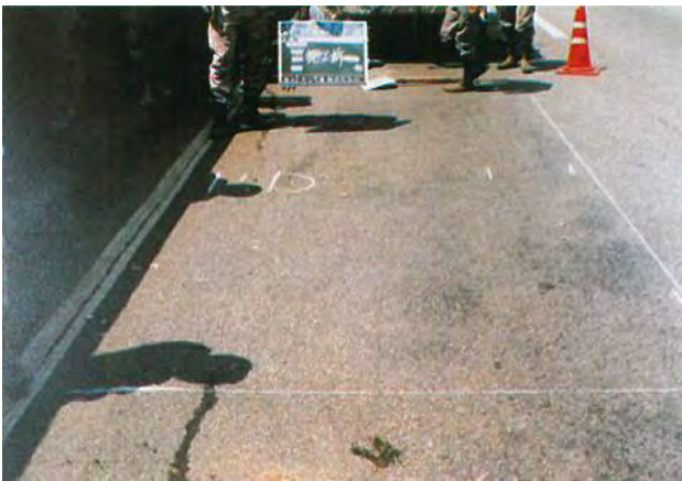
Photo 5.2.8.3 Pavement distress due to slab concrete damage
