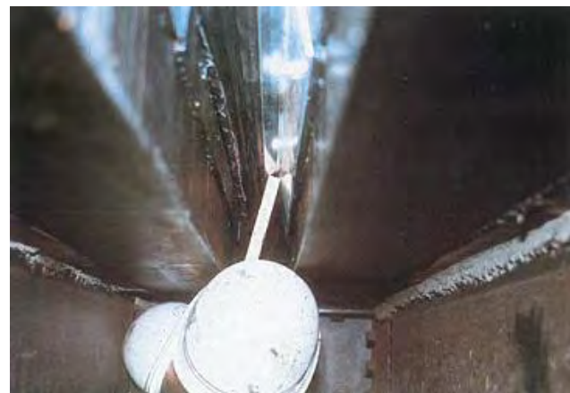
Photo 7.1.1.5 Installation of supporting metal pieces
