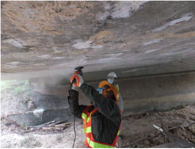
(a) To flatten by disk grinder
