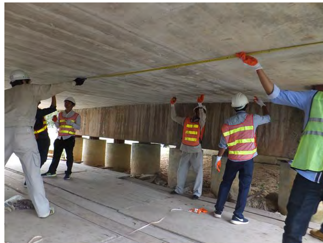
Photo 5.2.2.9 Measuring reinforce range
