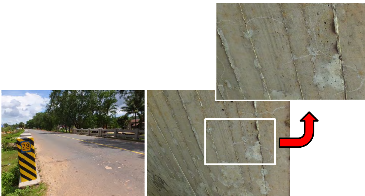
Photo 5.2.2.4 Concrete crack on slab
