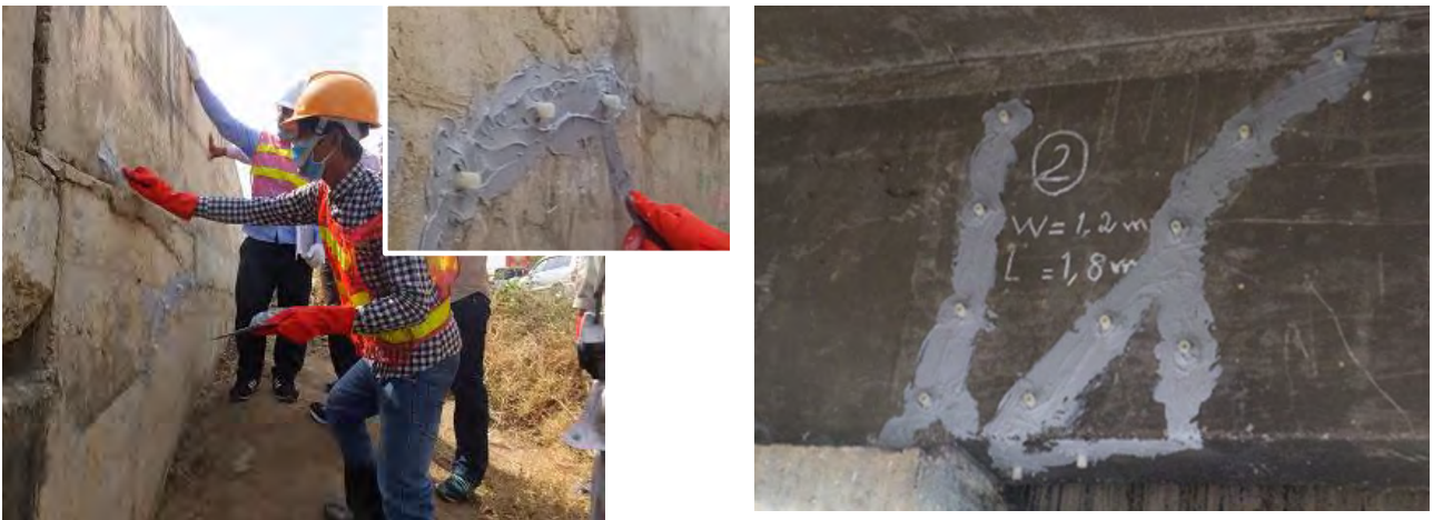
Photo 5.2.1.11 Attached Sealing on the crack
