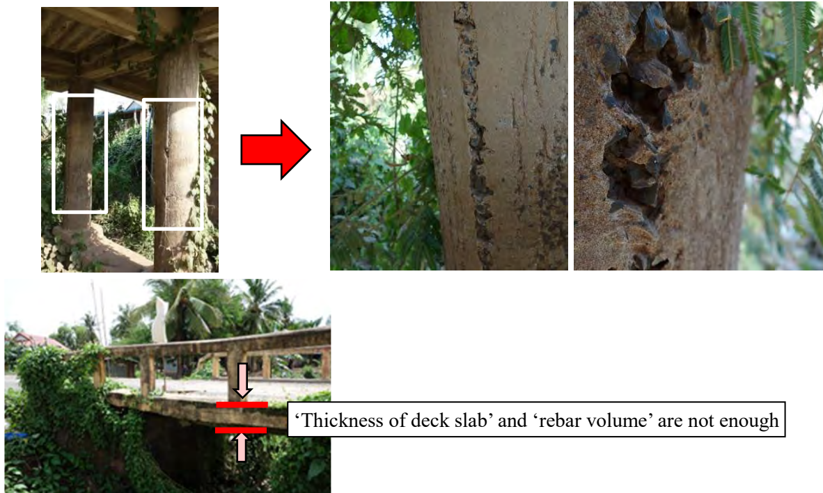
Photo 5.2.2.1 Insufficient strength capacity
