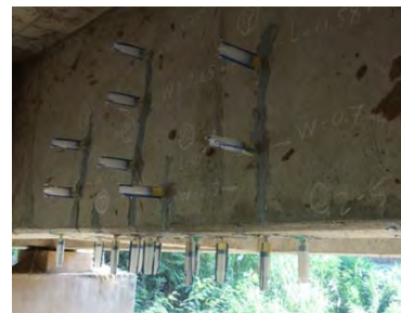
Remove syringes, washers and sealing
