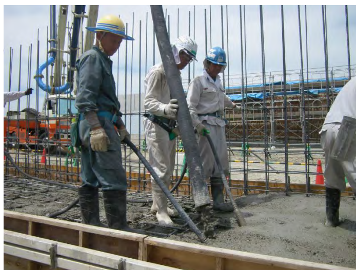
Photo 4.4.2 Compaction
