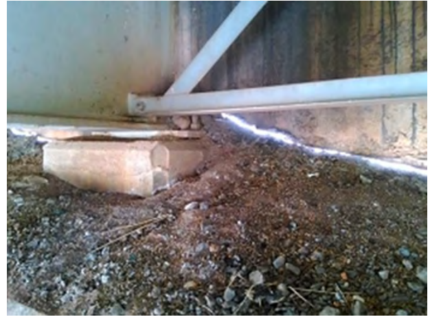
Photo 3.2.3.6 Mud, debris and sand deposits around Bearing seat areas
