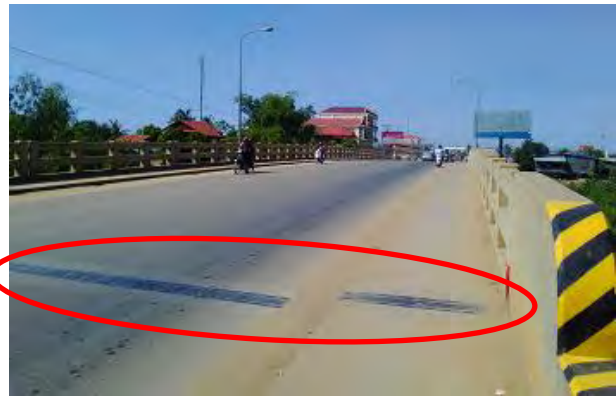
Photo 1.3.11 Expansion joint
