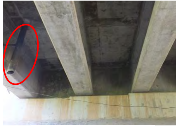
Photo 1.3.10 Drainage facility
