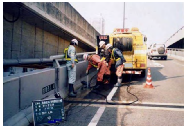
Photo 3.2.3.3 Drainage cleaning with water jet
