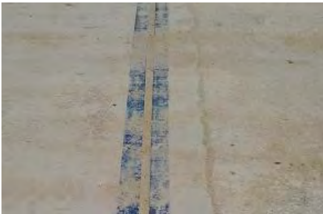
Photo 3.2.3.2 Expansion joint clogged with sand and dust
