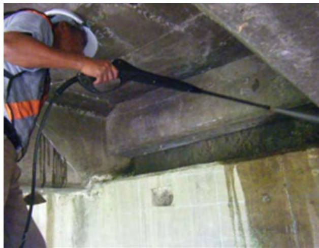
Photo 3.2.3.7 Cleaning of pier bearing seat
