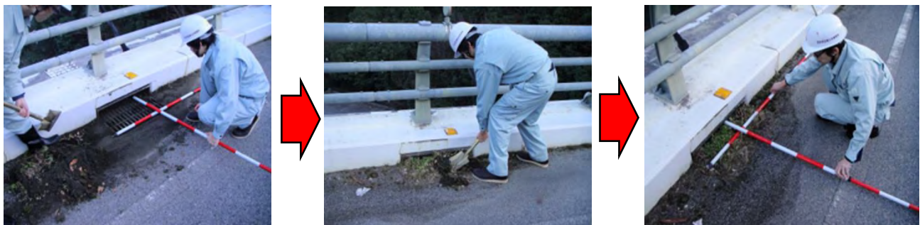
Photo 3.2.3.4 Manual drainage cleaning
