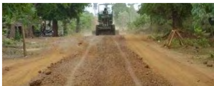
Figure-14 Grading for Unpaved Roads
