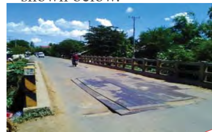
Disintegration around expansion joint
