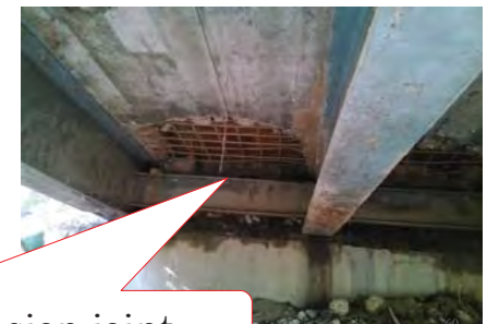
Disintegration around expansion joint
