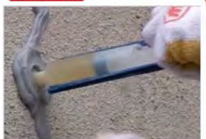
Injection into cracks with epoxy resin
