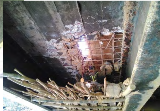
Phase 6 condition (disintegration)
