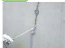
Remove syringes, washers and sealing
