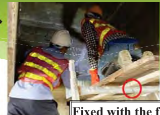
Fixed with the frame
