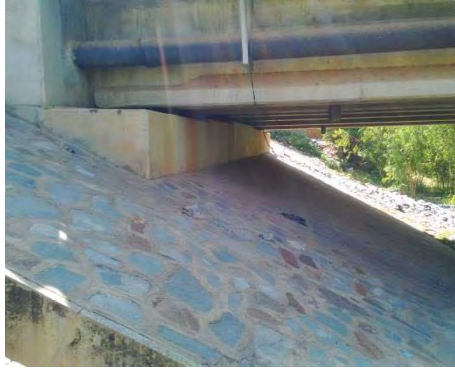
Protect from scouring (Left : RN2 Right: RN8) (Very good)
