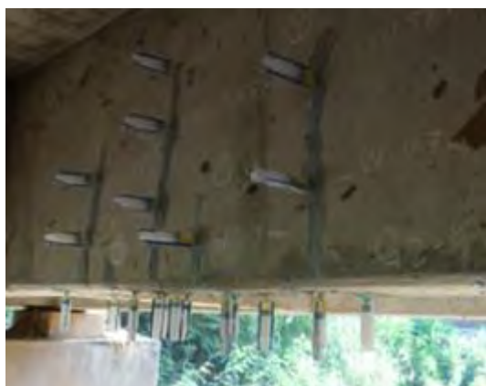
(a) Crack Sealing (1 st Pilot project)
