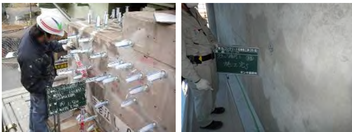
Photo 7-11 Concrete Crack Repair Method
