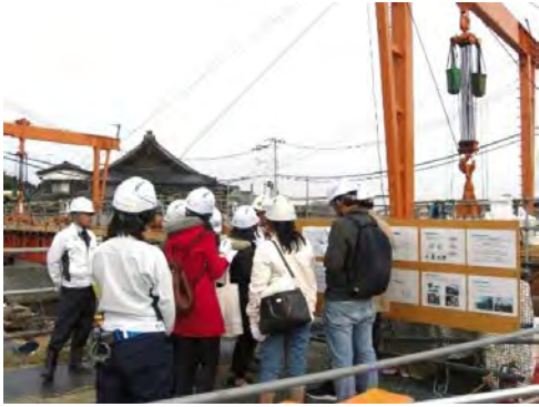
7 Nov Site visit of concrete bridge construction
