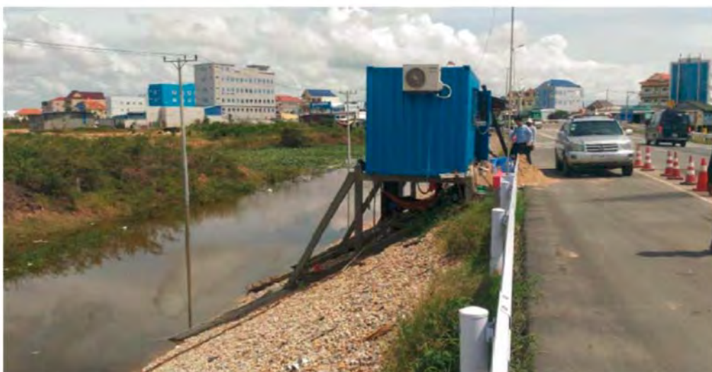
Operation House of East Neak Loeung Weigh Station
