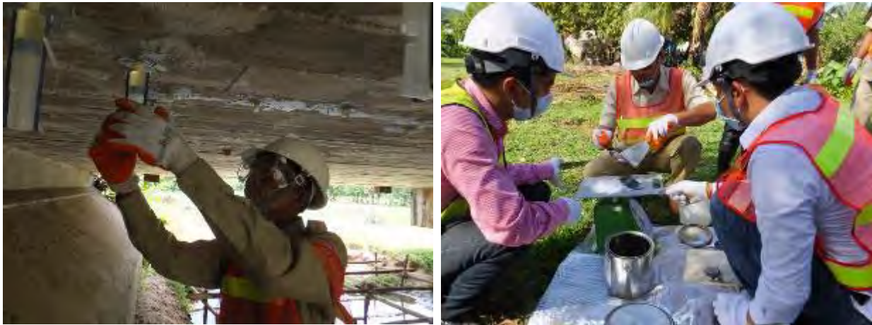
Figure 7-19 Crack Repair (Reference: 1 st Pilot Project)
