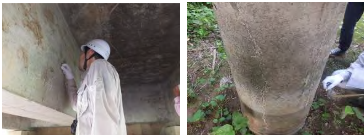
Photo 7-7 Field Survey for 1 st Pilot Project
