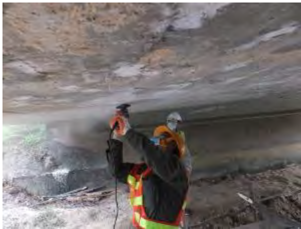
(a) To flatten by disk grinder
