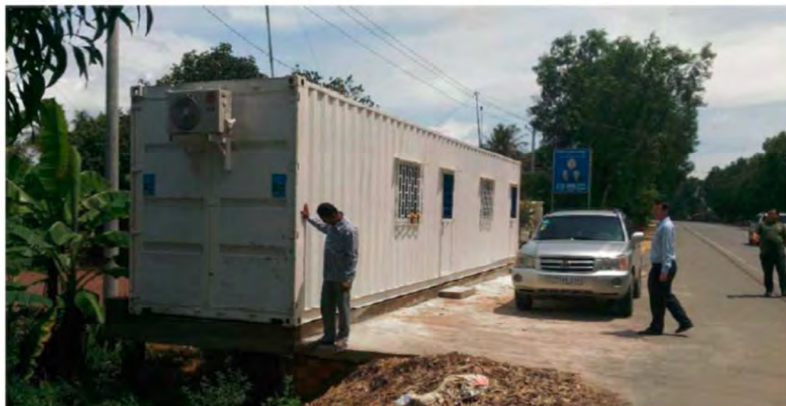
Operation Office of West Neak Loeung Weigh Station
