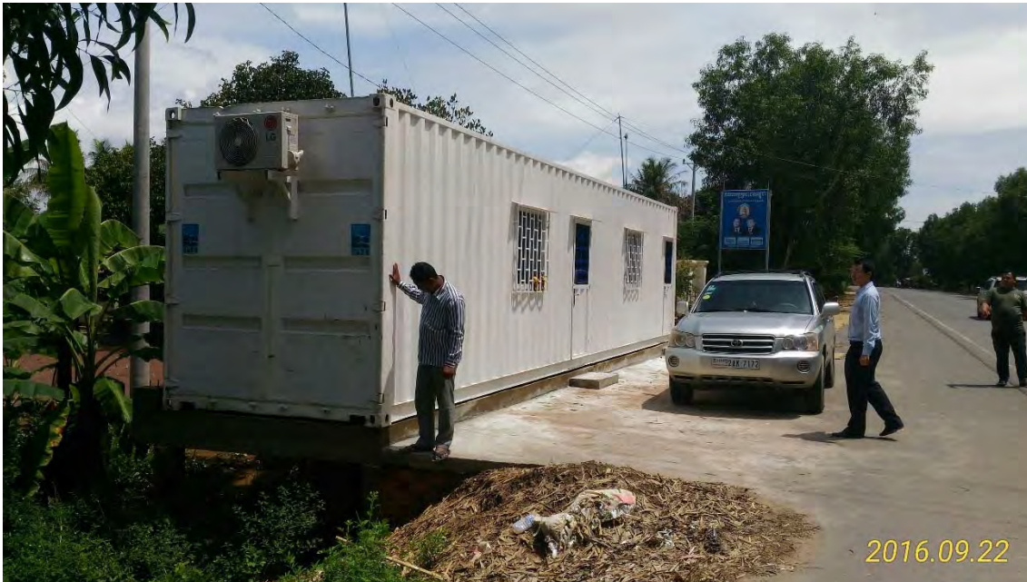
Container house west
