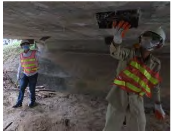
(b) To remove dust by polishing scrubbing
