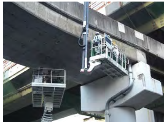
10 Nov OJT using bridge inspection car
