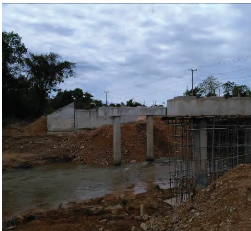
Sta.51+220 L=45m, W=8m
