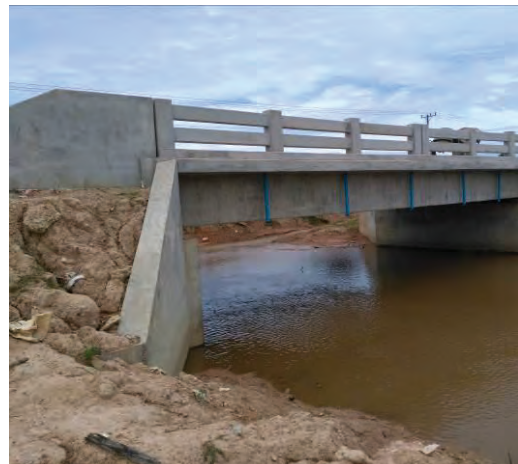
Sta.66+890 L=15M, W=8m
