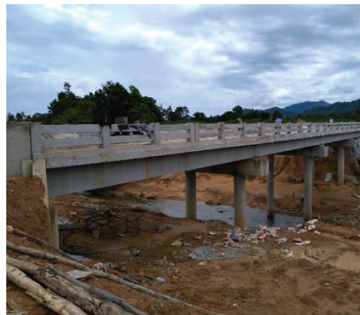
Sta.43+00 L=60m, W=8m
