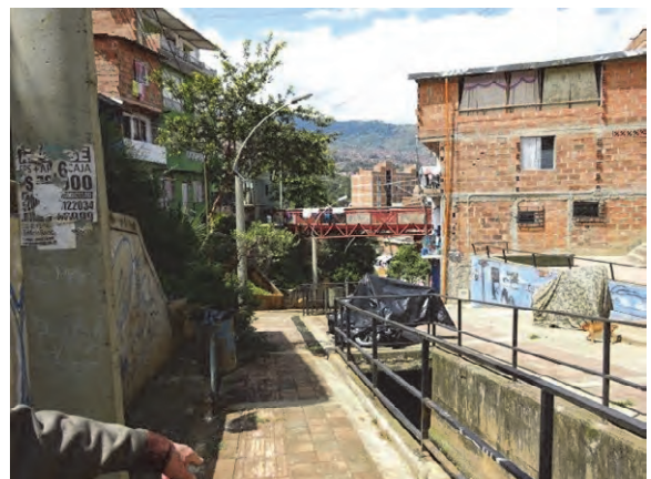
Pictured in the back of the photo is a newly constructed bridge, so as not to divide the residents on both sides of the mountain stream.
