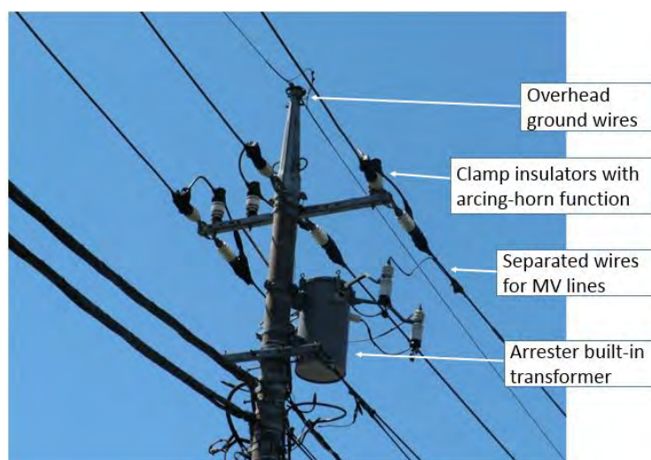
Figure 9-18 Typical distribution line in Japan
