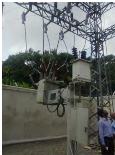
Figure 9-8 Auto Recloser Installed on the Gantry
