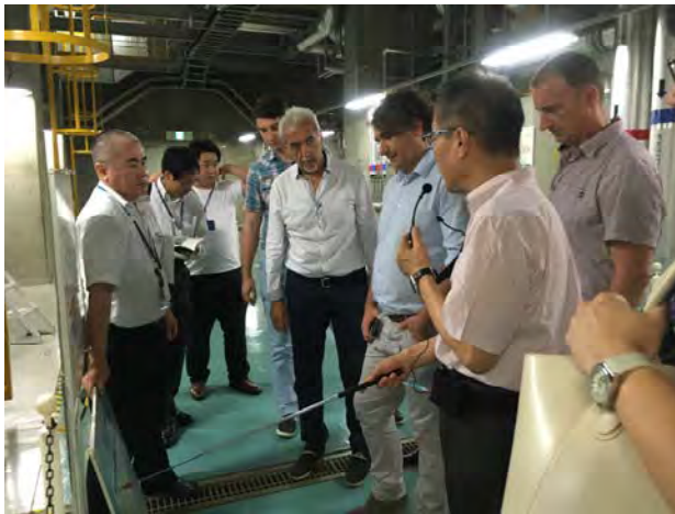
District Heating Plant (July 6) (Harumi Toriton Square)
