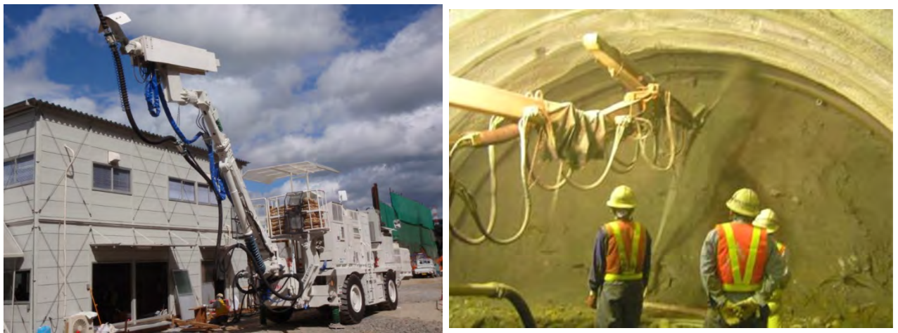
Figure 3-29 Shotcreting Machine (left) and Shotcreting (wet- process, right)
