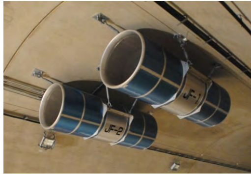
Figure 5-1 Attached Jet Fans (freely suspended type)
