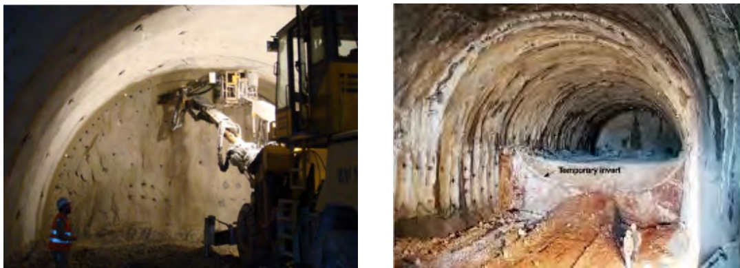
Figure 4-9 General Conditions of New Austrian Tunneling Method (NATM)
