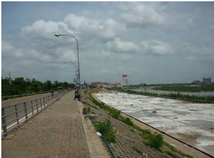
Figure 2.4.5: Flood control dike cum road along the Mekong River in Vientiane
