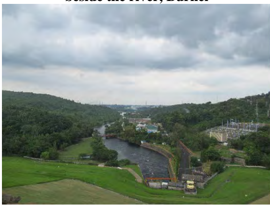
Downstream view from Jatilhul Dam Photo: JICA Project Team F5: Integrated operation of Jatilhul Dam, Indonesia
