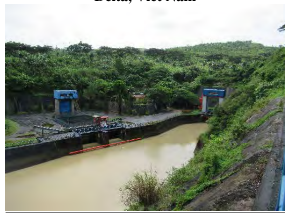
Neyama Tunnel (Inlet) Photo: JICA Project Team F6: Neyama Tunnel, Indonesia
