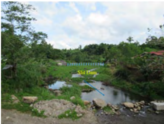
Slit Dam in the Anilao River Upstream Reach
