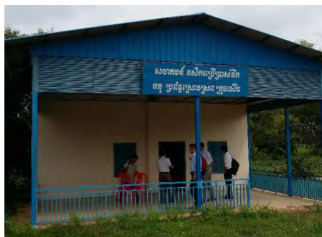
Figure 3.5.6: Office of a water user association in Cambodia
