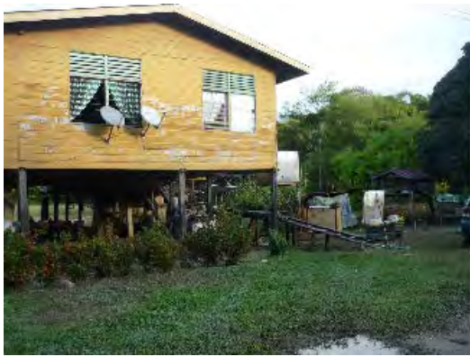
Elevated house Photo: JICA Project Team F3: Elevated house in flood prone area beside the river, Burnei
