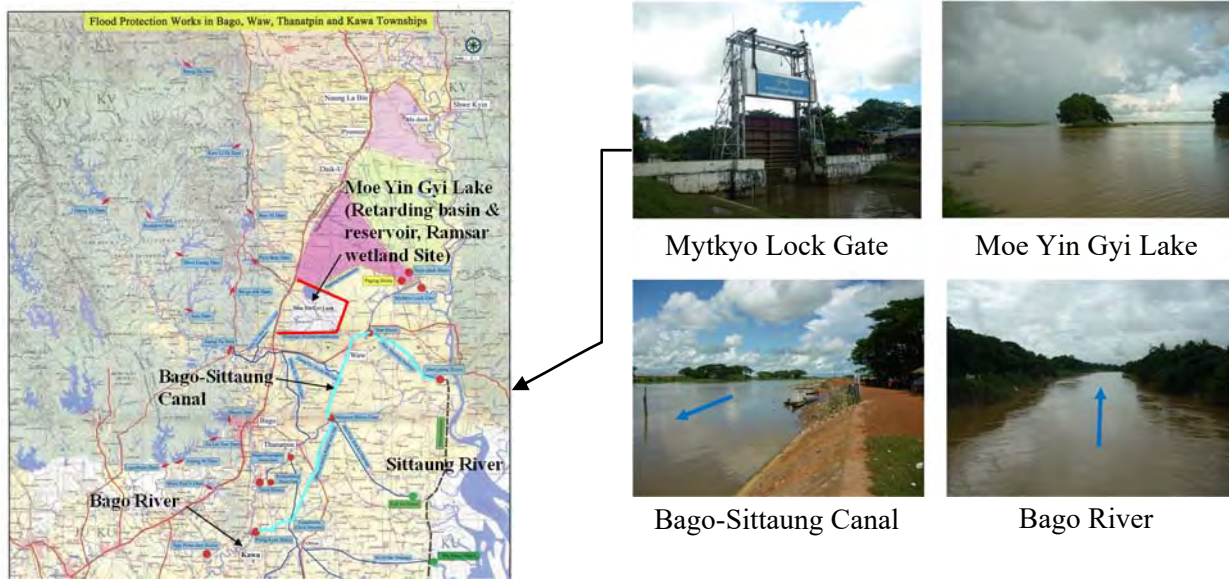
Figure 2.6.3: Bago river flood control and navigation channel system Source: IWUMD (Irrigation and Water Utilization Management Department: map) and JICA Project Team (photos)
