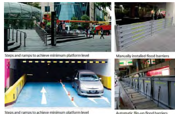
Figure 7. Examples of flood prevention measures. From "Managing Stormwater for our future" by the PUB, Singapore's National Water Agency (PUB). (2014)
