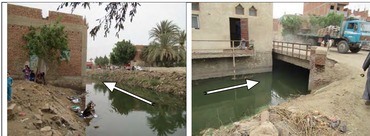
Interpenetrated structure (mosque) inside Kella canal ( affects the hydraulic performance)
