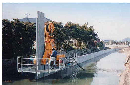
Figure 6.4 Implant Method
