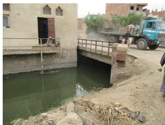
Figure 4.45 Malfunction of Water Flow and Control Caused by a Building (Mosque)
