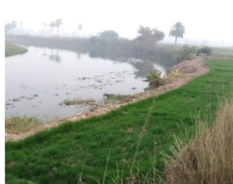
Protection work washed out at peak of flow rate. (Dlhans Bridge village)
