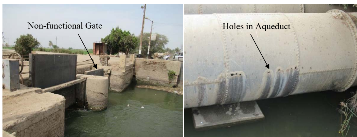
Figure 4.42 Aged Irrigation Facilities(Regulator and Aqueduct)
