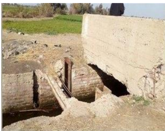
Figure 4.48 Naga Canal Intake of Damat Branch Canal (Gate Breakage)
