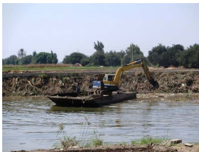
Figure 4.53 Dredging of Principal Canal
