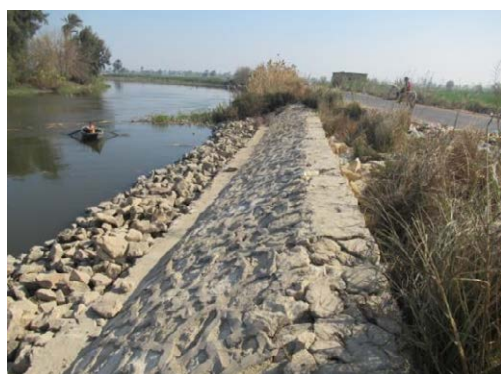
Protection work constructed by MWRI. (Around El Gafadon village)
