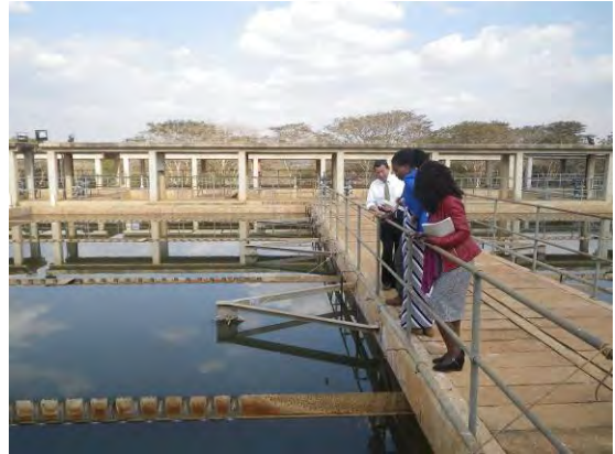
Water Treatment Plant LWB WTP (Jul.18, 2017)
