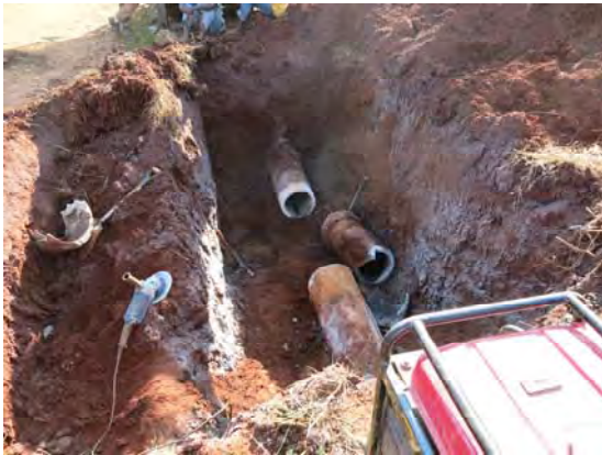
Leakage Prevention Work Lilongwe Sounth Zone (Jul.26, 2017)
