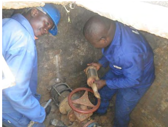
Water Pressure Meter Exchange Work Lilongwe South Zone (Jul.27, 2017)
