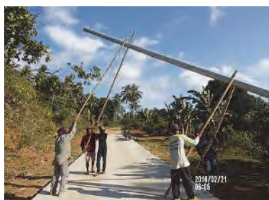
Manual Pole Installation Work
