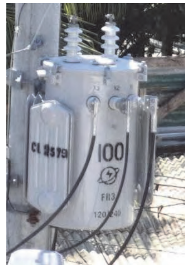
Figure 2-2.1 Pole Transformer
