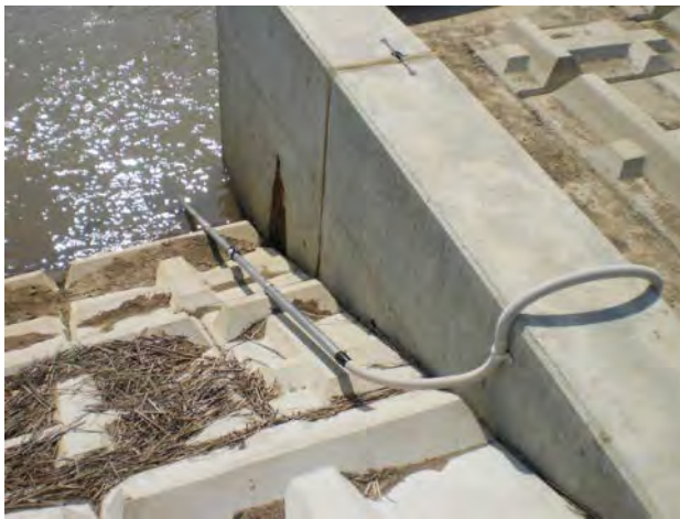
Example of combination with measuring instrument (water gauge)
