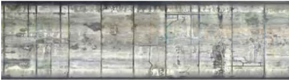
Cavity inspection inside a tunnel
